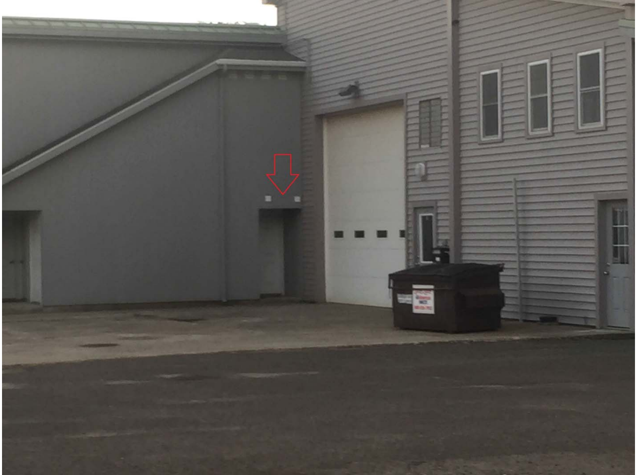
FIGURE 3 – 318 New Haven Avenue. Rear of building. Receiving/delivery door marked.
