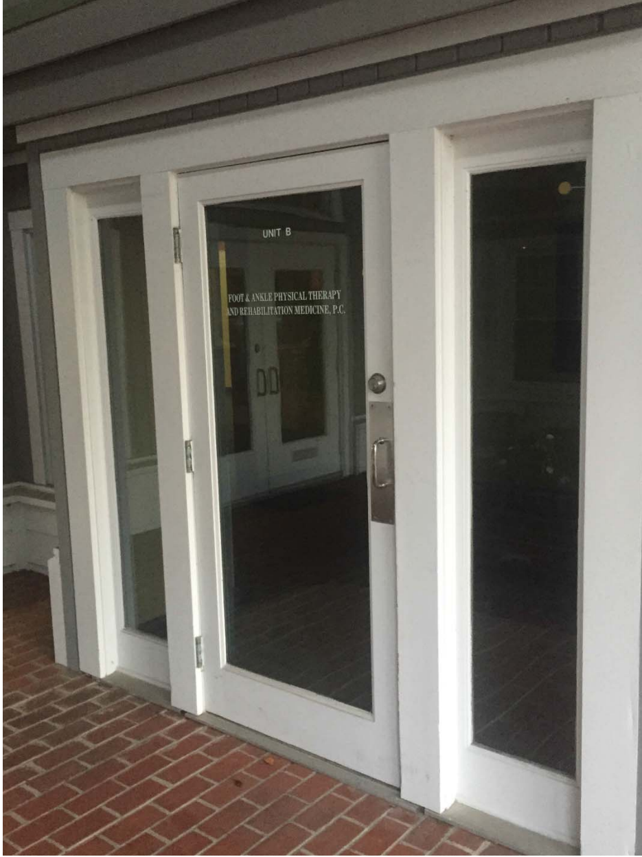
FIGURE 4 – 318 New Haven Avenue. Door to Unit B.
