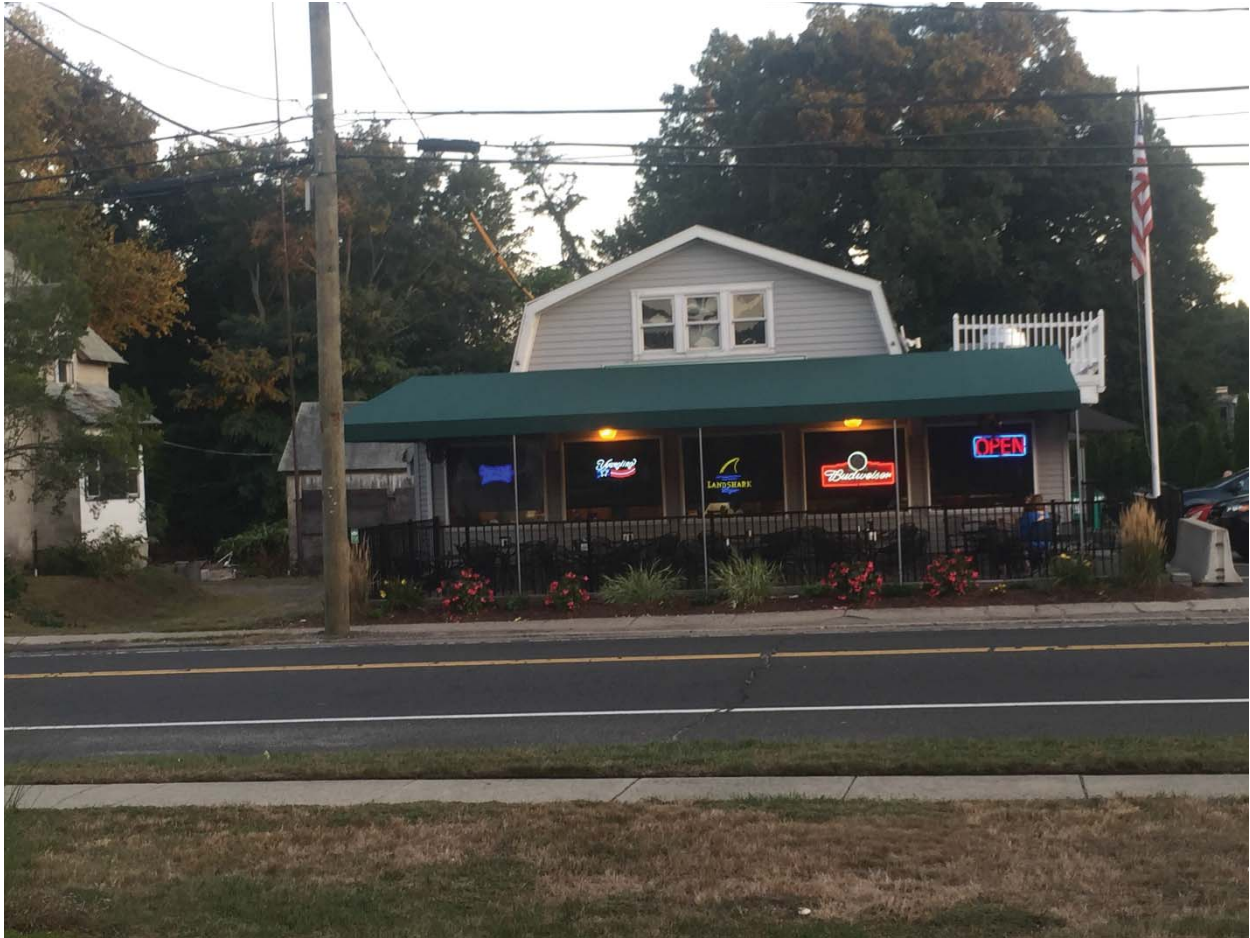
FIGURE 8 – New Haven Avenue. Restaurant directly across street from property.
