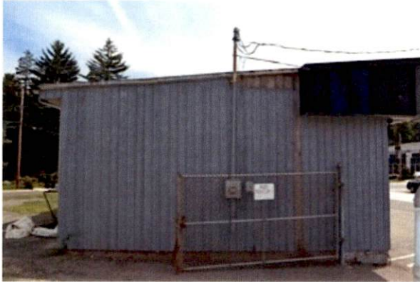
Photo 4: Left side of the dispensary facility.
