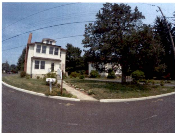
1. Split Family Home 7 & 9 Roller Terrace, Milford, CT 06460.
