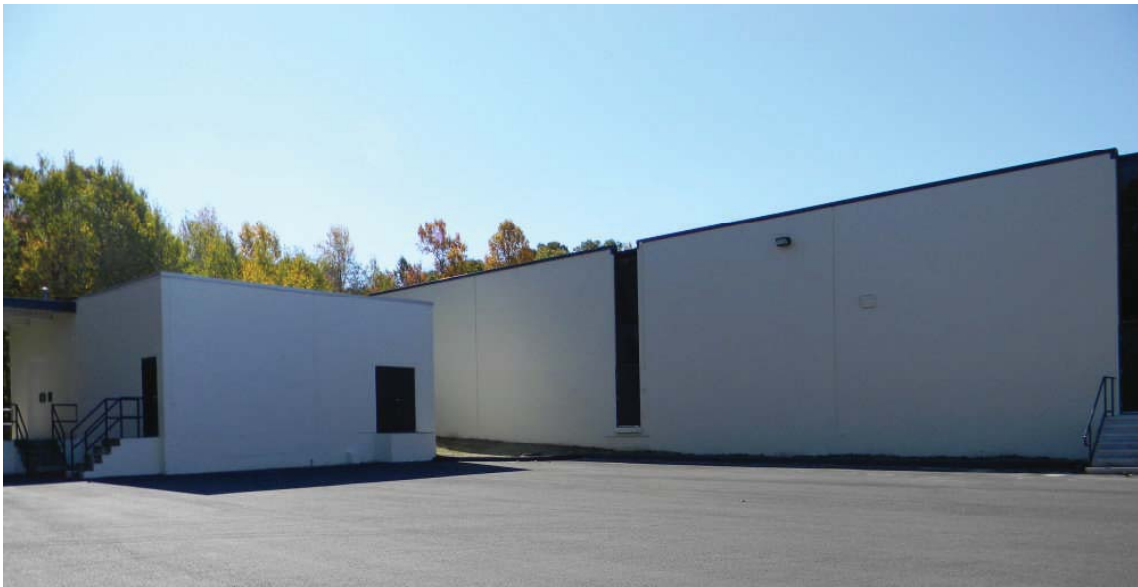
400 Captain Neville Drive (Initial 30,000 sq ft Production Space and Office Annex)
