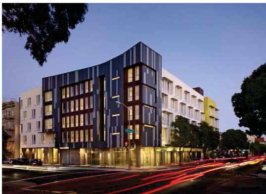
Drs Jullian and Raye Richardson Apts. San Francisco, CA David Baker Architect, Photo Credits: Bruce Damonte
