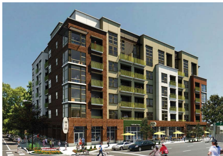
16 Powerhouse, Sacramento, CA D&S Development LPA Sacramento
