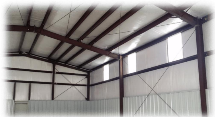
Conventional X-Bracing
