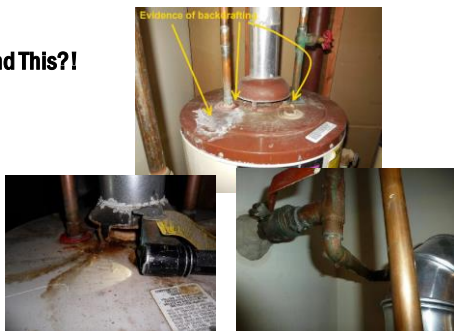
...Unenforced/ Badly Detailed Energy Code Requirements!!! - MAJOR Cause of CO Poisoning/Death!
