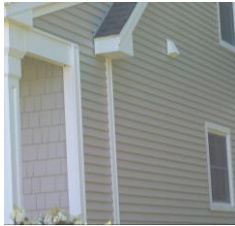
Exhaust opening for Range hood
