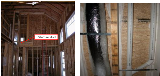
Return air duct built into wall for second and first floor
