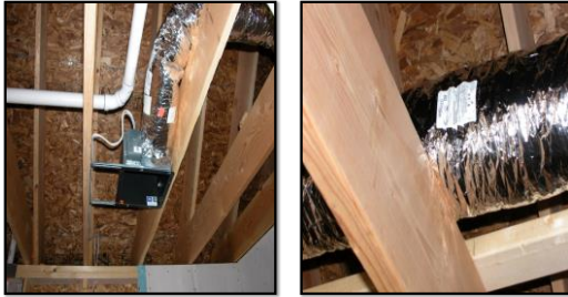
Duct for second floor bath fan
