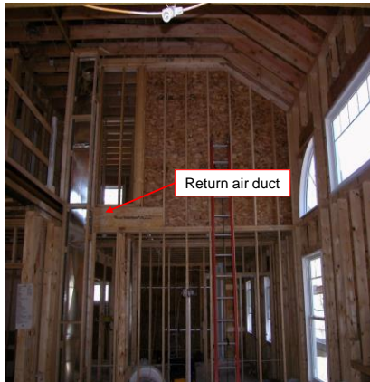
Return air duct built into wall for second and first floor
