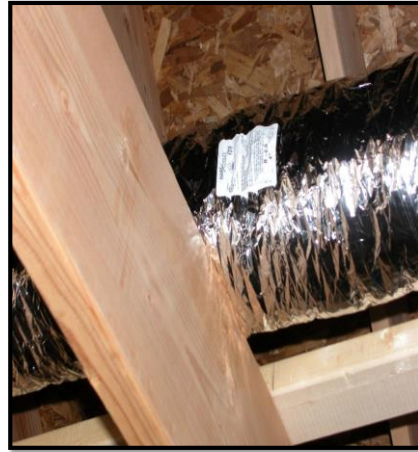
Duct for second floor bath fan
