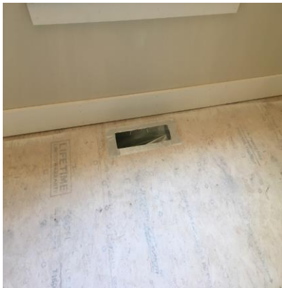
Typical duct floor termination
