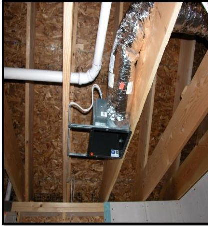
Duct for second floor bath fan
