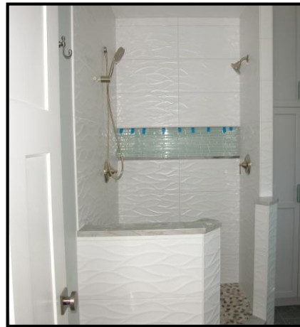
Almost finished master bath shower area
