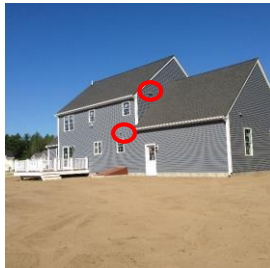
This Home has 2 Bath Fans Both Rated to Operate at 80 CFM
