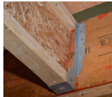
Hanger Restrains Top Flange
