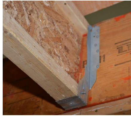
Hanger Restrains Top Flange
