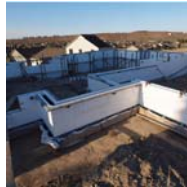
Insulated from top of basement wall down to 10 ft below grade or basement floor, whichever is less
