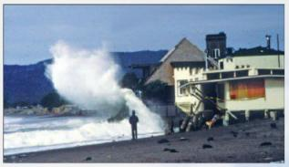
deflection, and wave uplift. The most severe damage is caused by breaking waves (see Figure). The force created by waves breaking against a vertical surface is often 10 or more times higher than the force created by high winds during a storm event.
