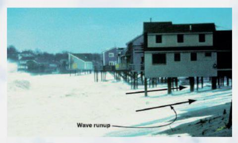
Wave runup occurs as waves break and run up beaches, sloping surfaces, and vertical surfaces. Wave runup (see Figure 3-24) can drive large volumes of water against or around coastal buildings, inducing fluid impact forces (albeit smaller than breaking wave forces), current drag forces, and localized erosion and scour (see Figure).
