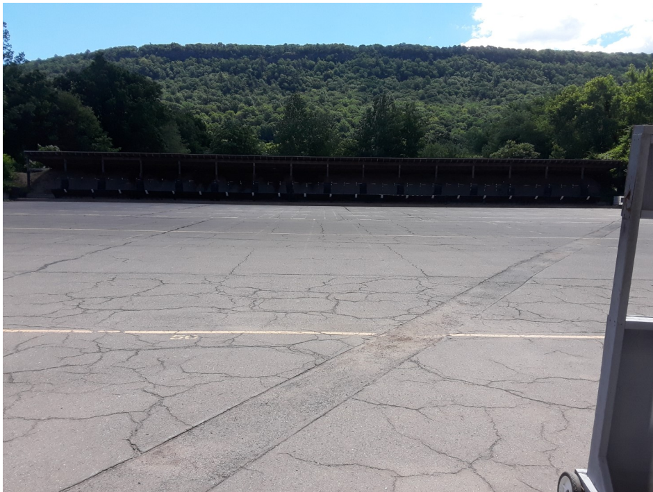
Figure 4-1: Pistol Deck Paving
