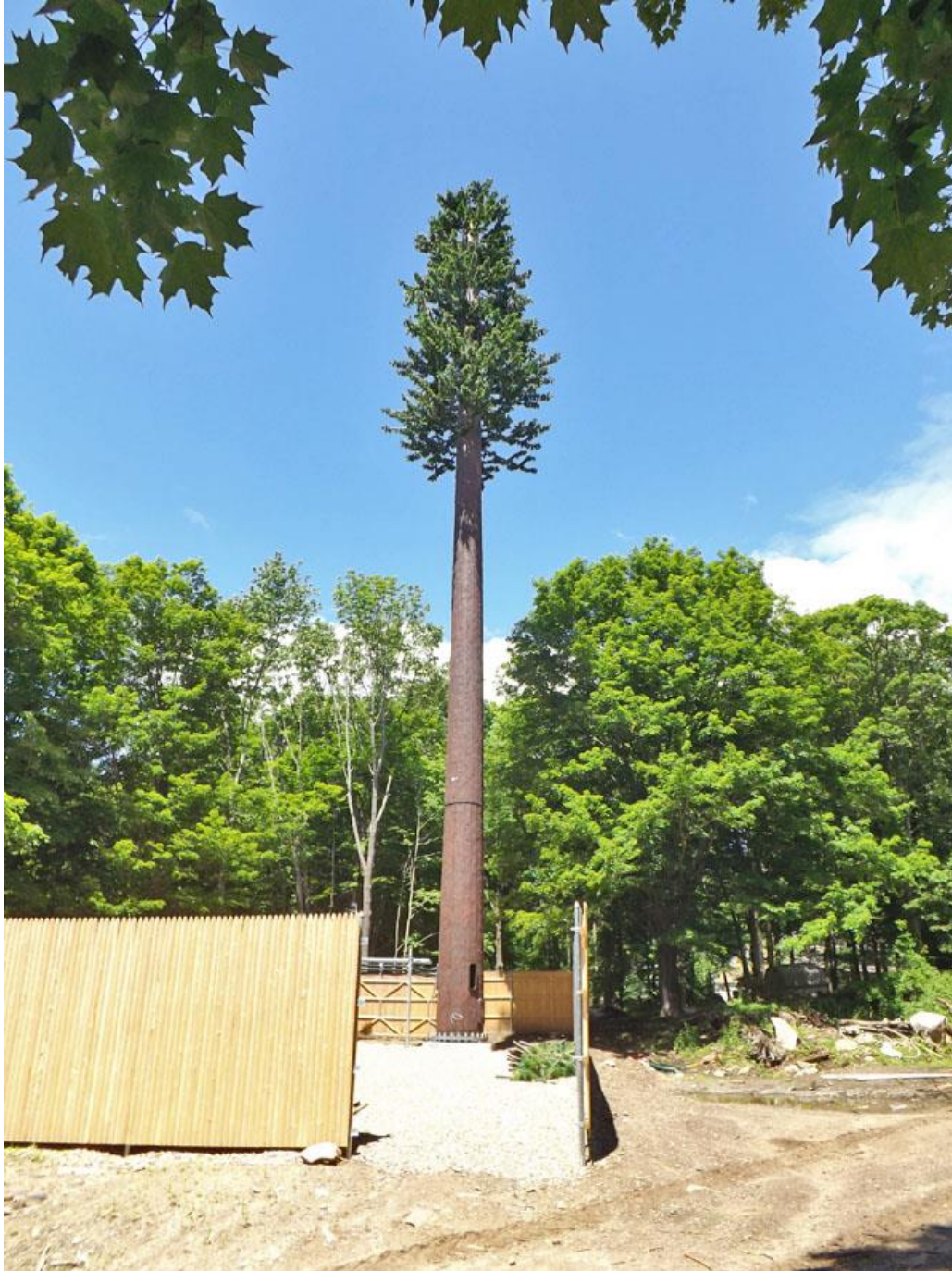
View of tower
