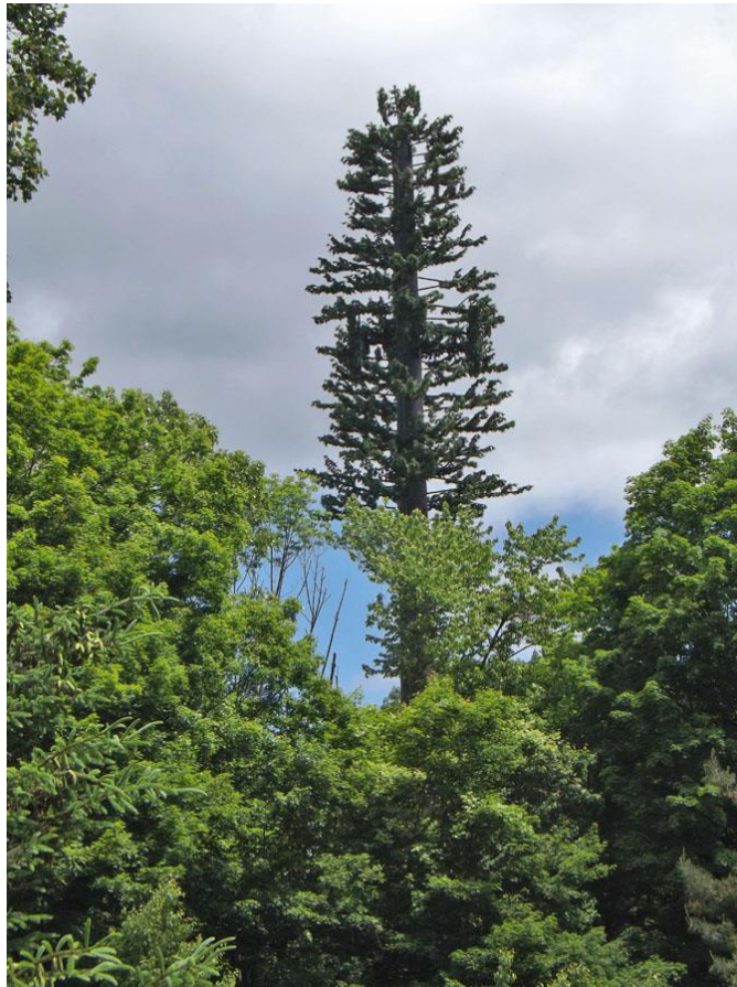
View of tower from access road
