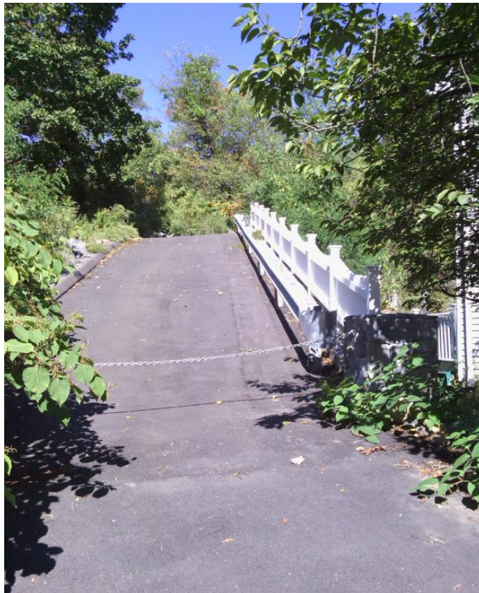
Access Drive extending from Ritch Avenue. Property to left (east) is 42 Ritch Avenue (Hartwell).
