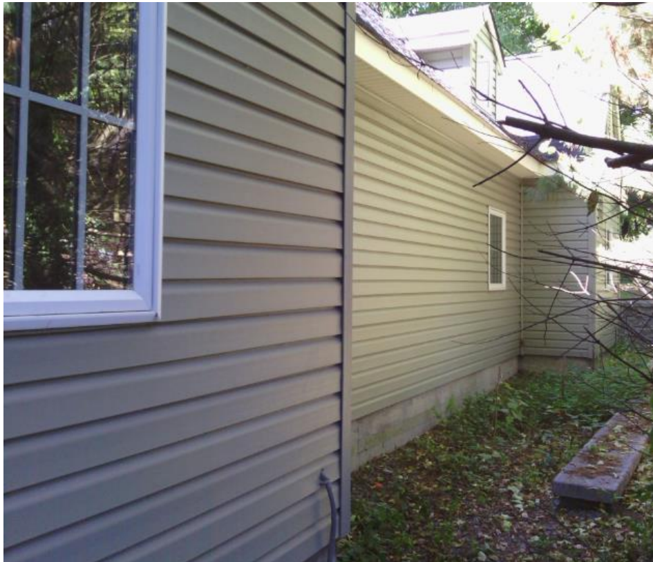
East side of compound/building wall. Property line to right.
