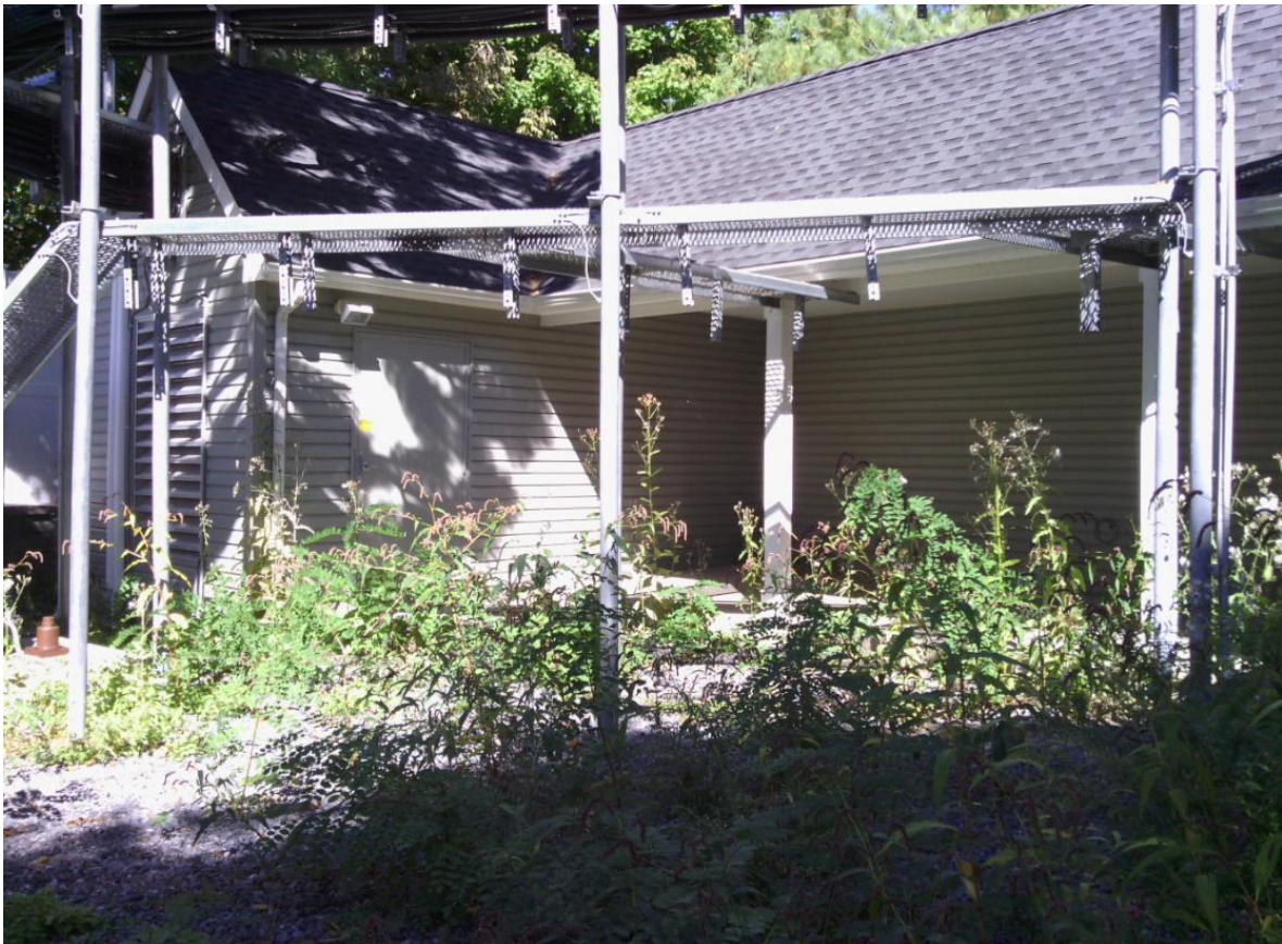
Interior compound area. Note weed growth.
