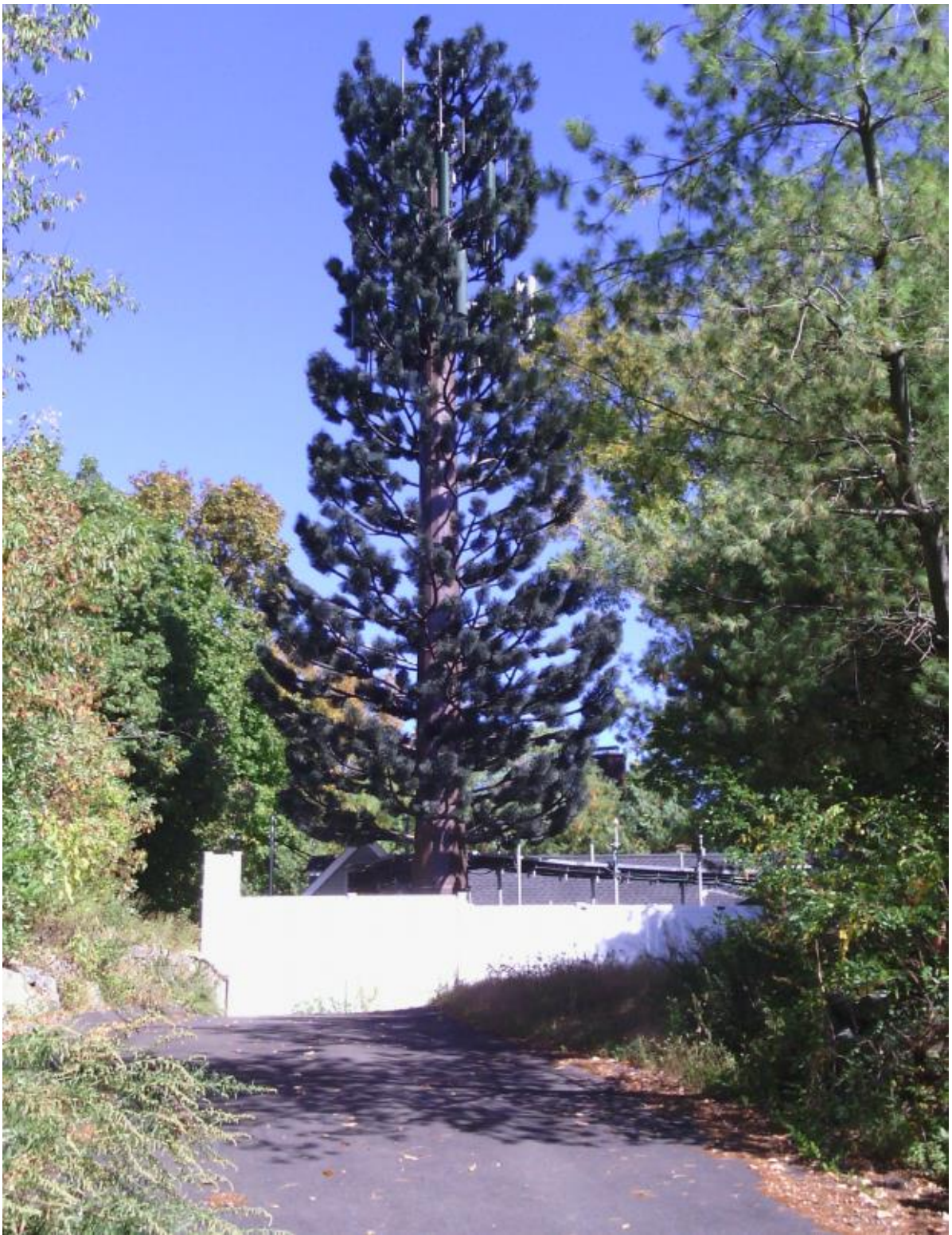
Compound view from access road as it reaches plateau above 42 Ritch Avenue.
