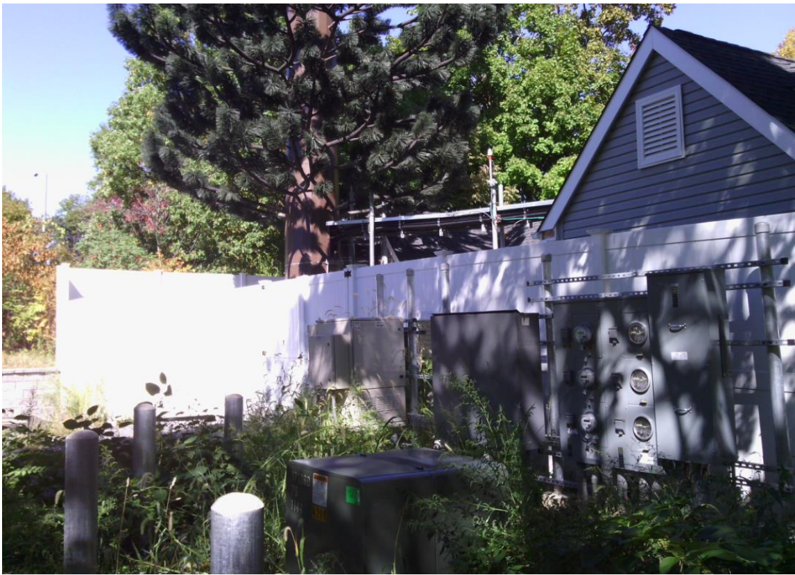
View from compound parking. Note weed growth.
