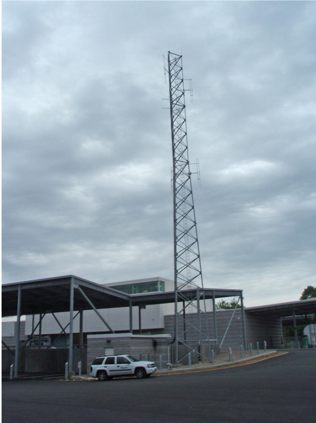
View of tower
