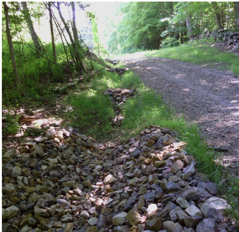
Check dams and ditch protection along access road.
