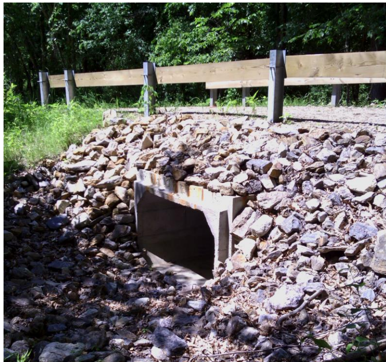
Box culvert outlet protection.
