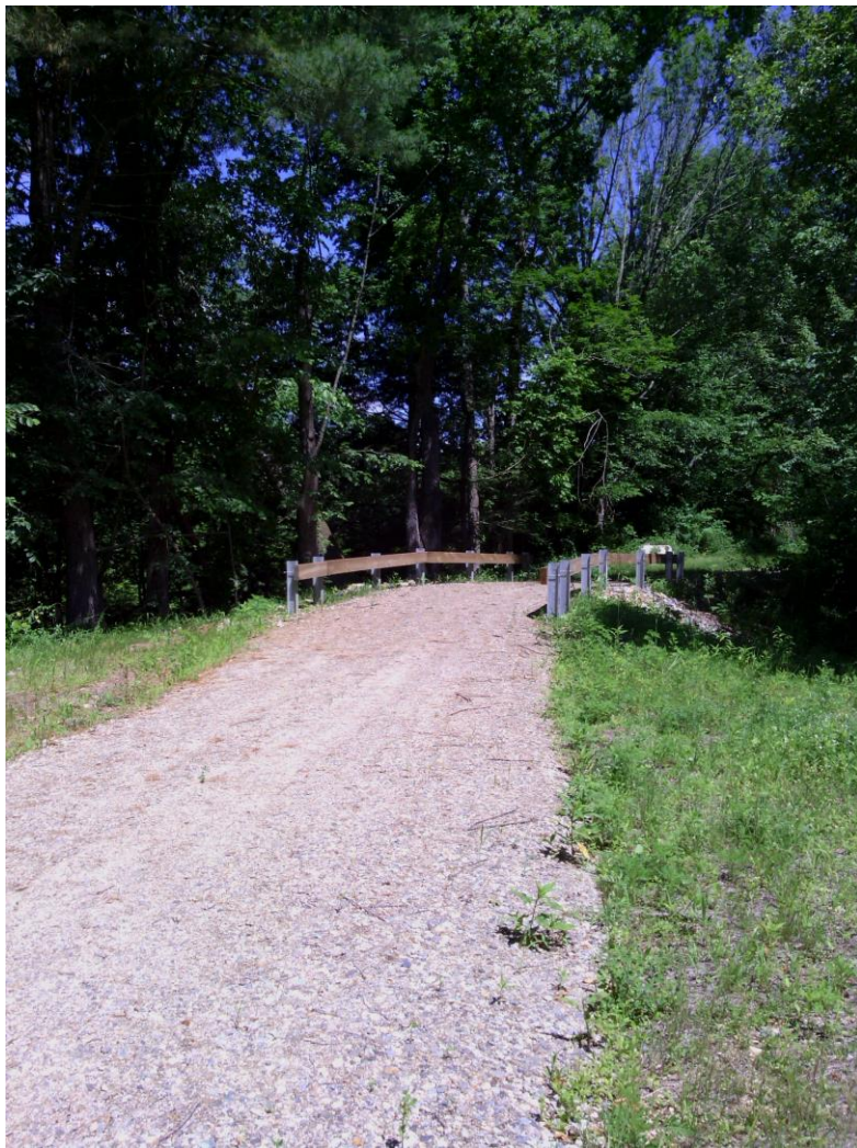
Access road over box culvert
