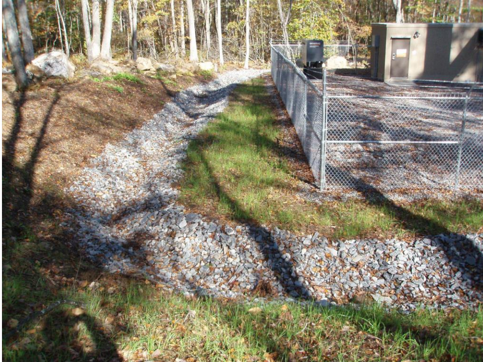
Riprap swales around perimeter of equipment compound
