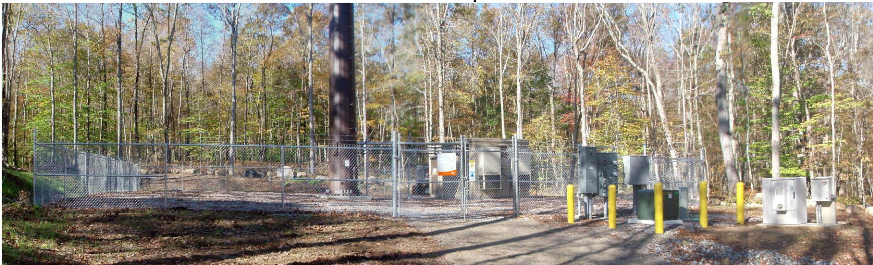
View of base compound
