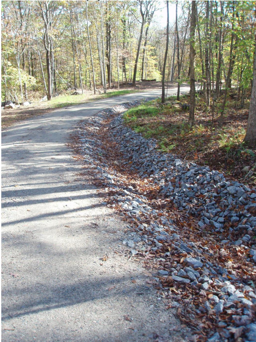
Riprap swale along access drive
