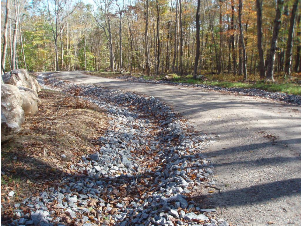
Riprap swales adjacent to access drive
