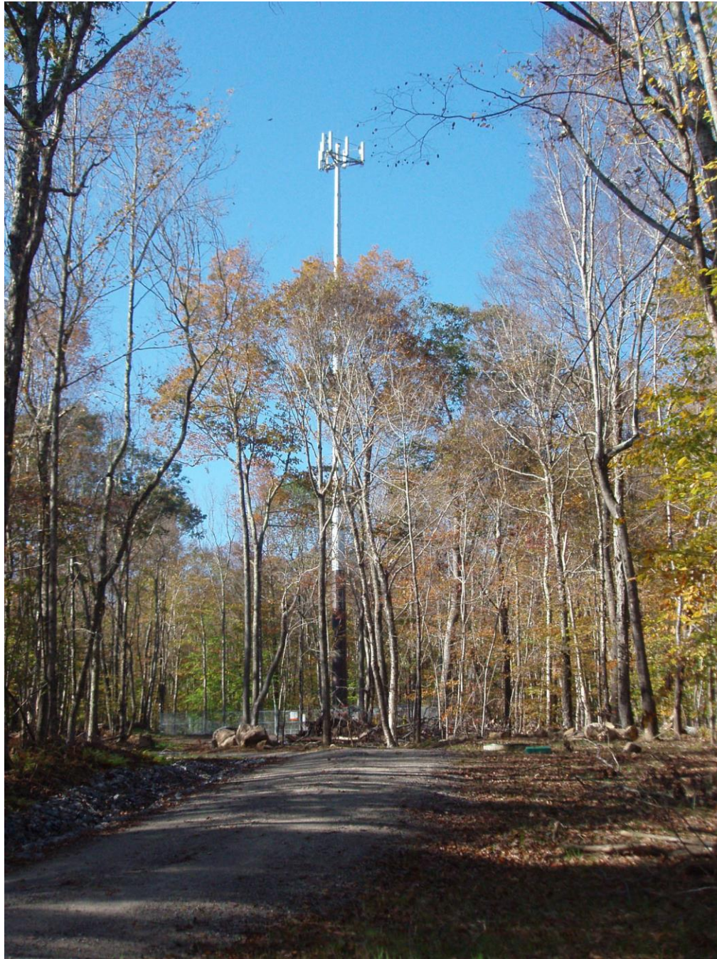
View of tower
