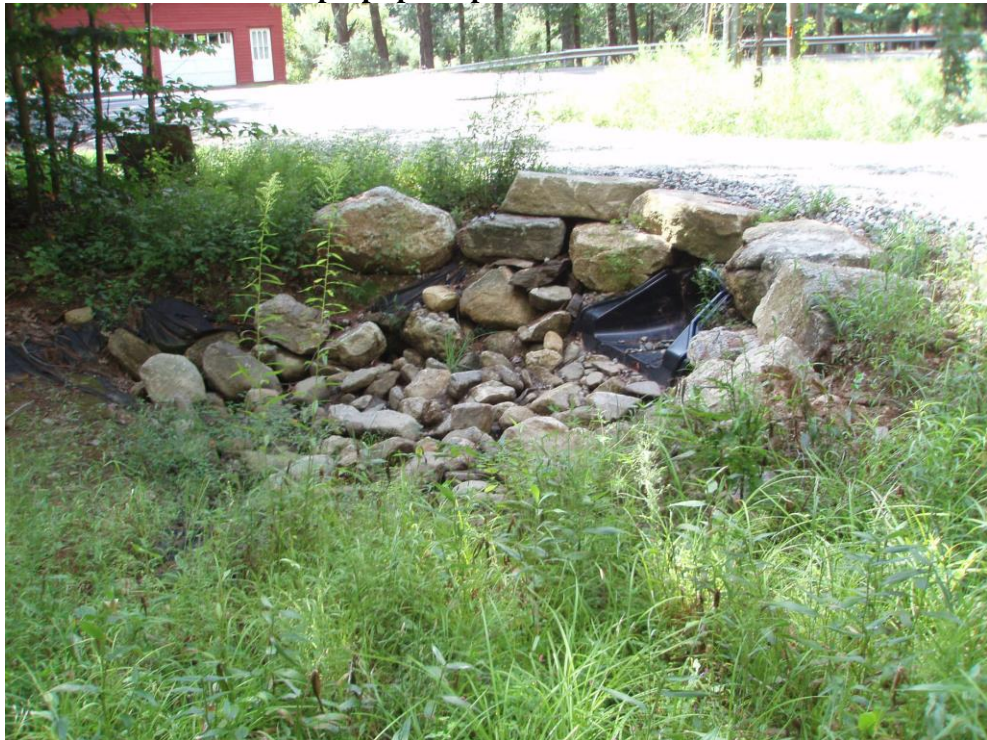
Culvert and riprap splash pad near access drive entrance
