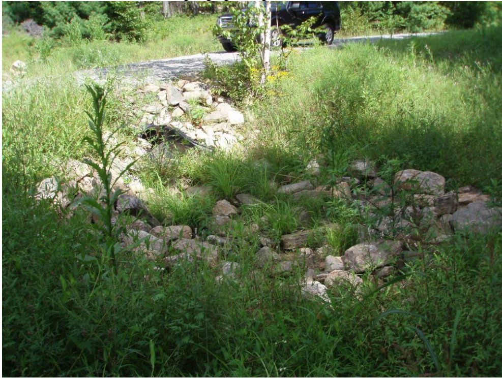
Culvert and riprap splash pad near access drive entrance
