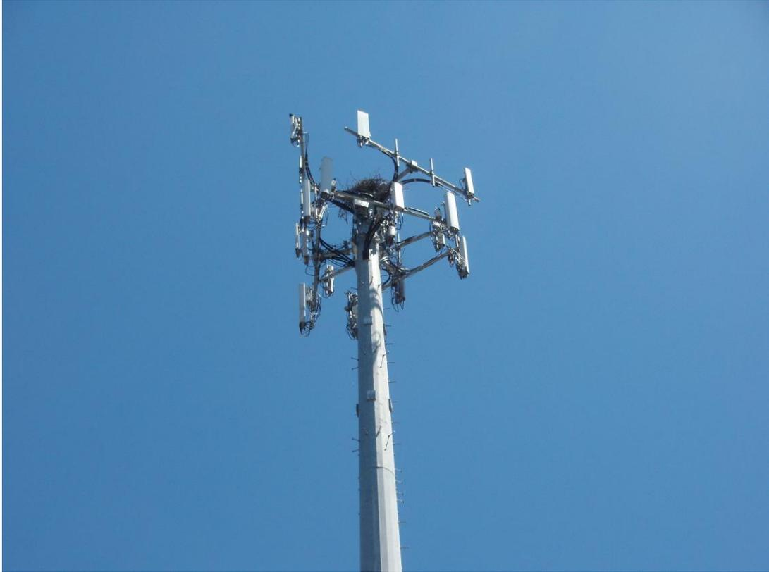
Antenna configuration - T-Mobile at 123 feet. AT&T at 112 feet. Note bird nest at top of tower.
