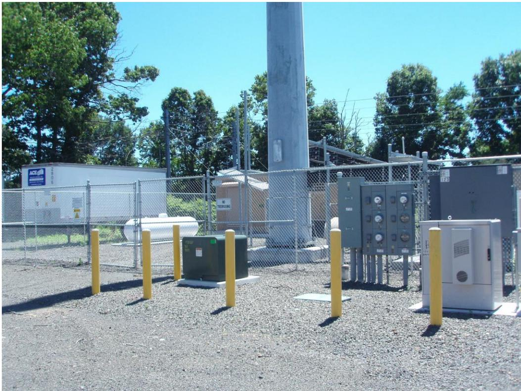
Utility board with bollard protection.
