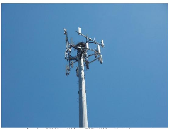
Antenna configuration - T-Mobile at 123 feet. AT&T at 112 feet. Note bird nest at top of tower.
