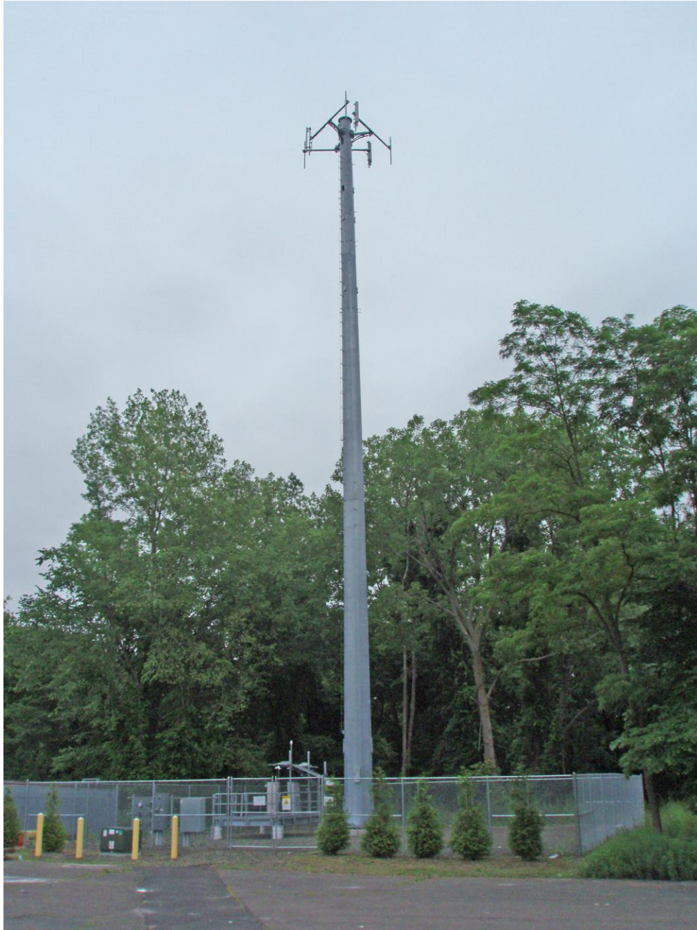
View of tower
