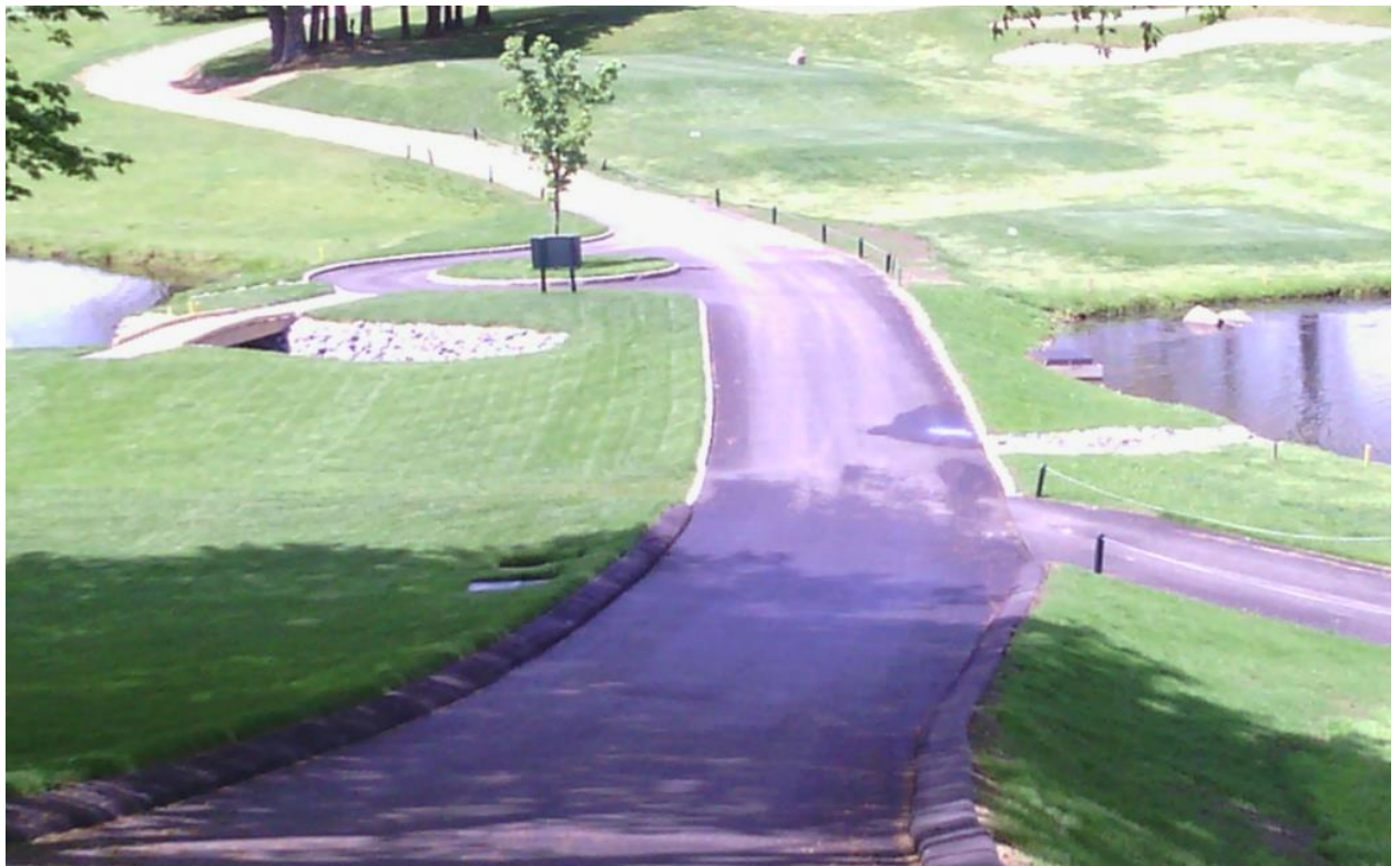
Access Drive/Golf Path along 11 th fairway. New culvert with rip-rap.
