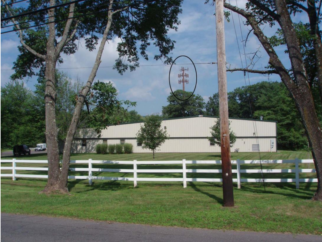
View of tower from across Burr Street
