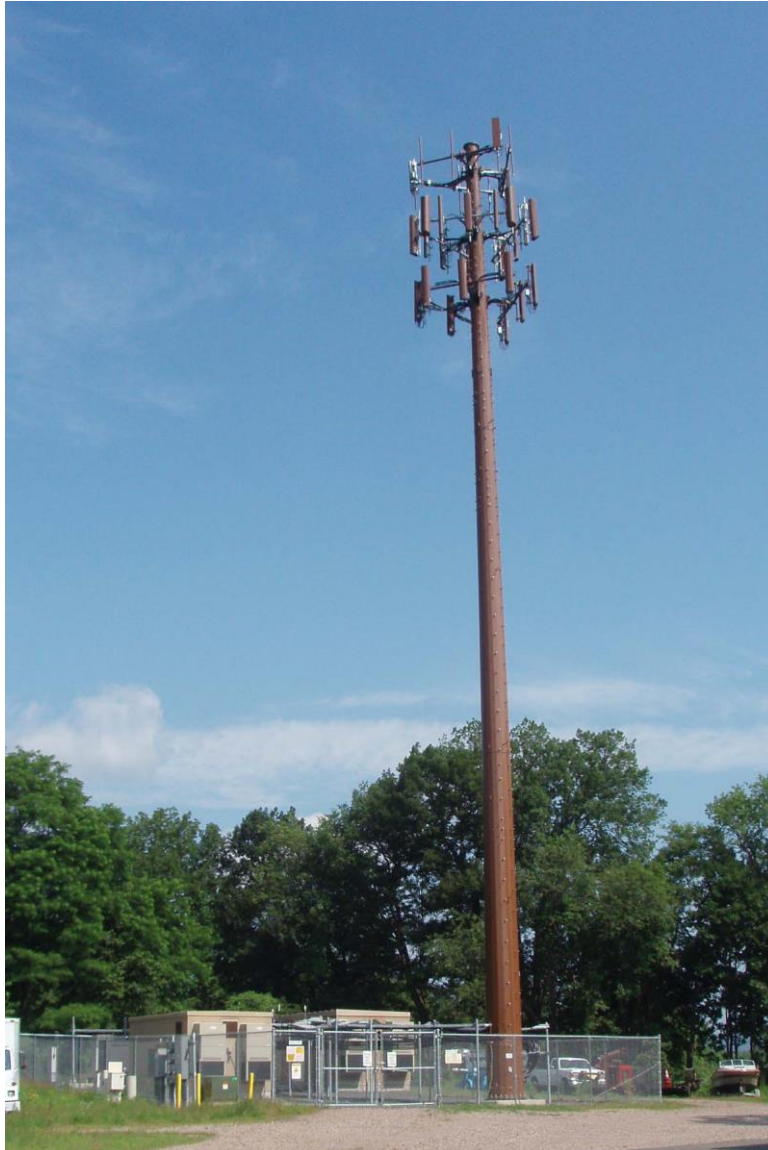
View of tower
