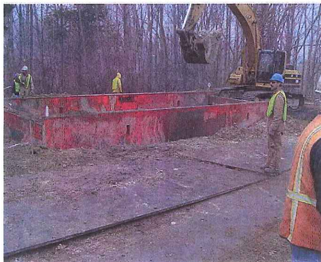
Figure 2-1: Typical 345 kV XLPE Splice Vault (Under Construction)
