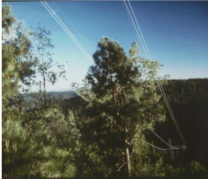
Figure D-1: Danger tree in transmission ROW
