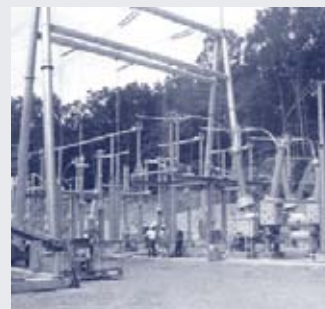
Figure 5.1 Archers Lane 345-kV Transition Station ( While Under Construction)
