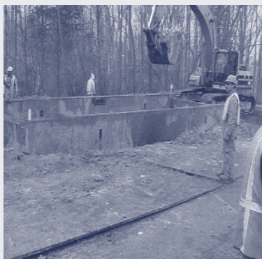
Figure 3.1. Typical 345 kV, XLPE Splice Vault (While under construction)
