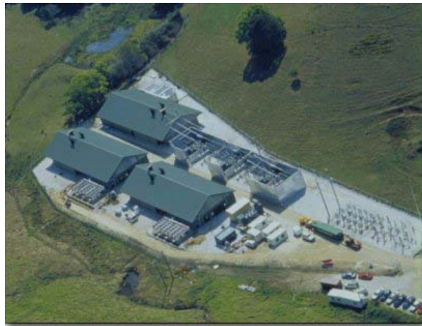
Figure 23 Three 60-MW Directlink converters working in parallel
