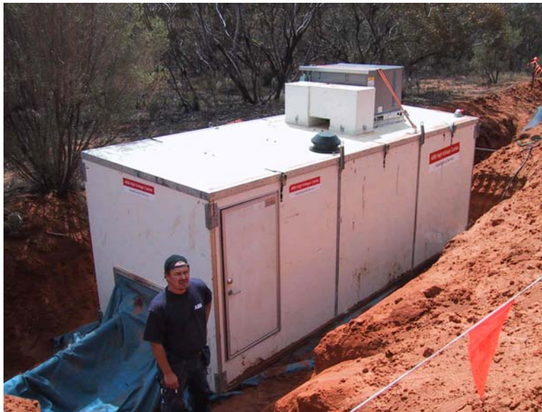
Figure 22, Jointing container, placed above the cables during jointing at Murraylink.
