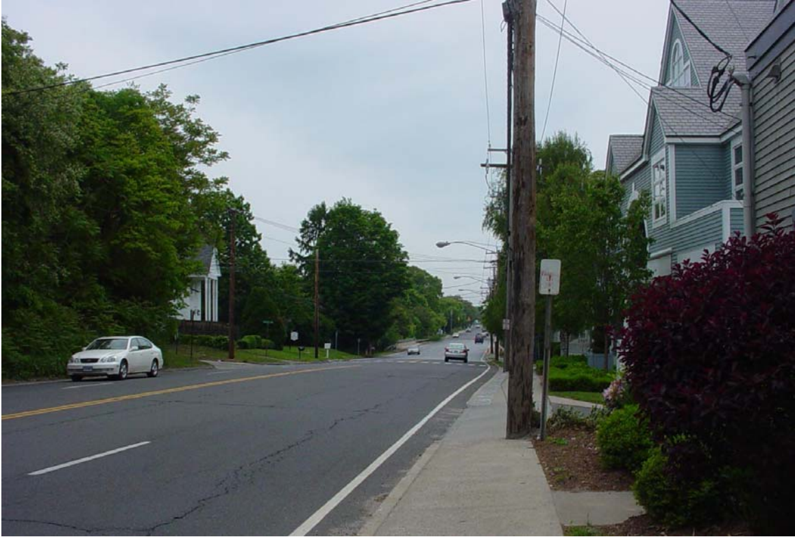
Photo 14. Route 1 (Post Road) looking eastbound west of Lacey Place.
