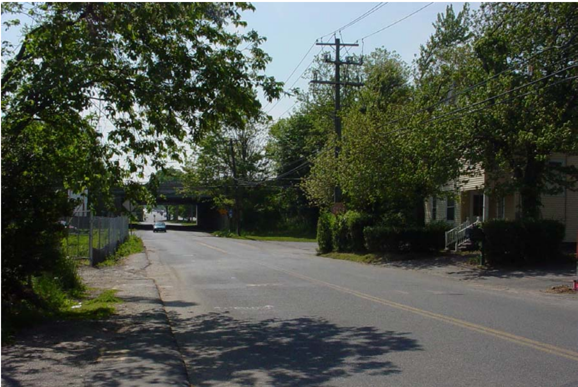
Photo 6. Old Post Road looking northwest toward the Interstate 95 overpass, east of Rennell Drive. Vertical clearance is sub-standard at 13'-9".
