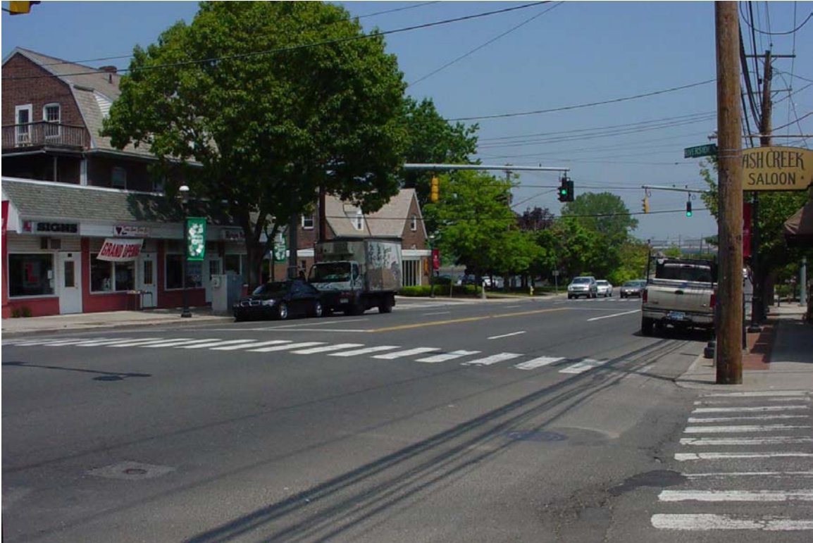
Photo 22. Route 130 looking eastbound at Riverside Drive.
