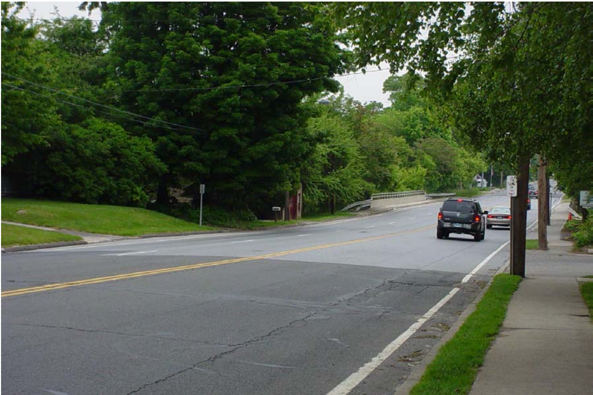
Photo 15. Route 1 (Post Road) looking eastbound west of Southport Harbor Bridge.
