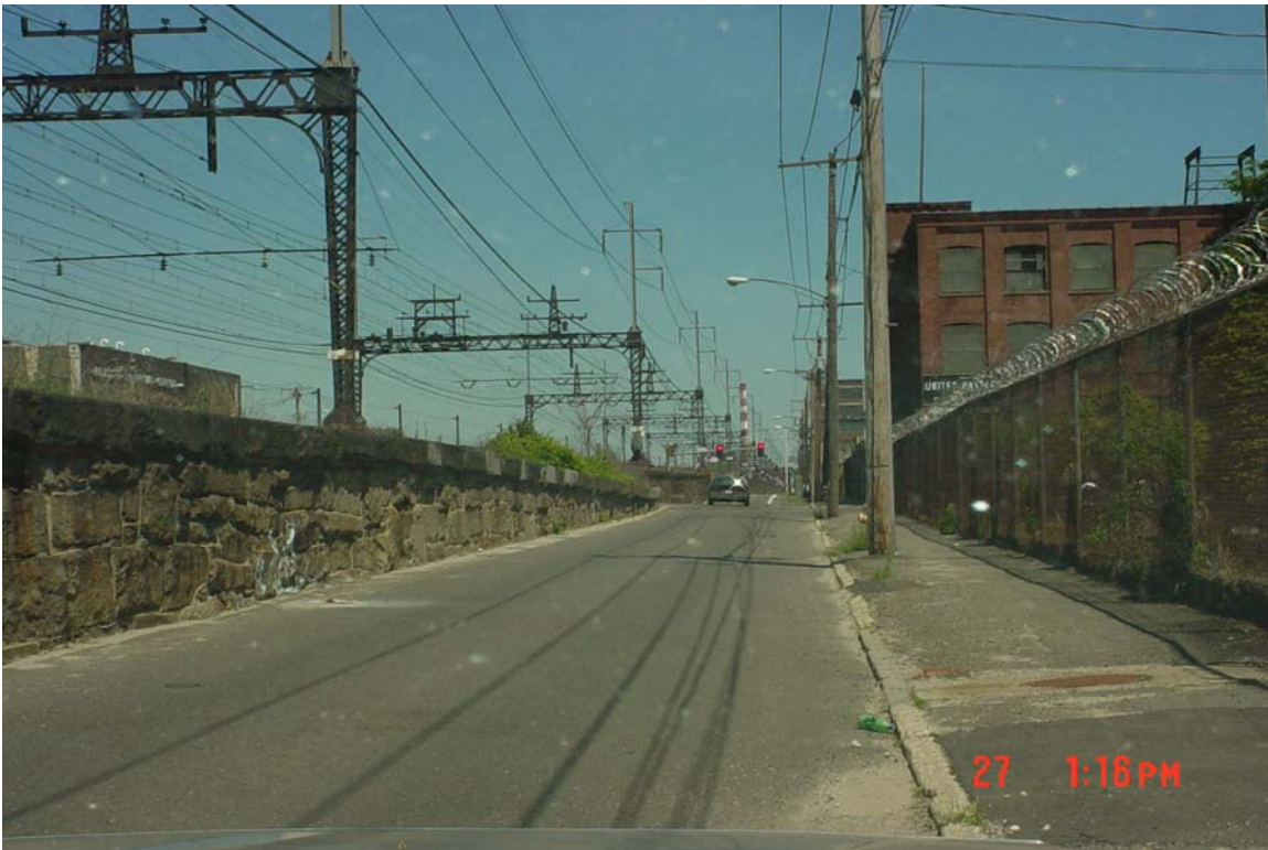
Photo 7. Railroad Avenue (EB) looking eastbound toward Bostwick Avenue. The roadway width in this area is approximately 17 feet.
