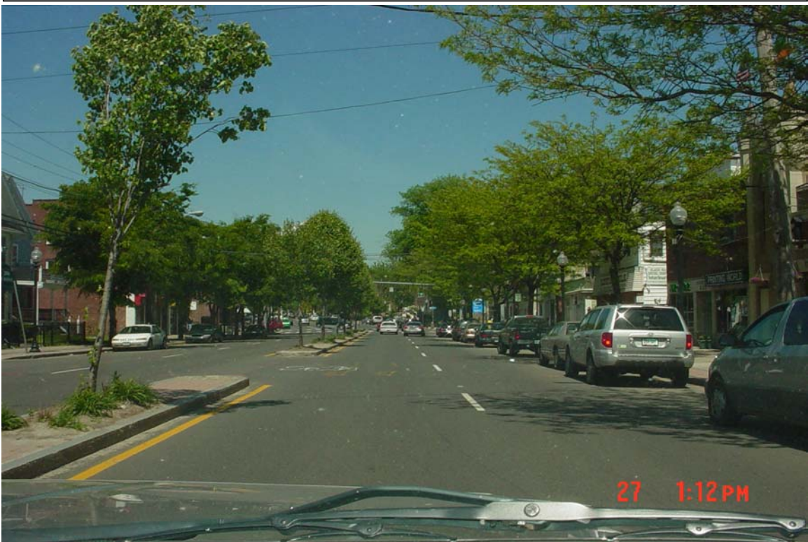
Photo 2. Route 130 (Fairfield Avenue) looking northeast between Jetland Street and Brewster Street. Notice the raised streetscaped median and on-street parking.
