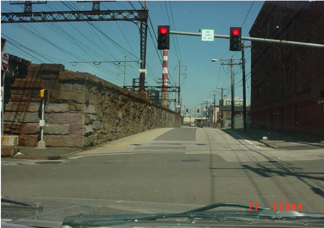
Photo 12. Railroad Avenue (eastbound) looking east at Myrtle Avenue.
