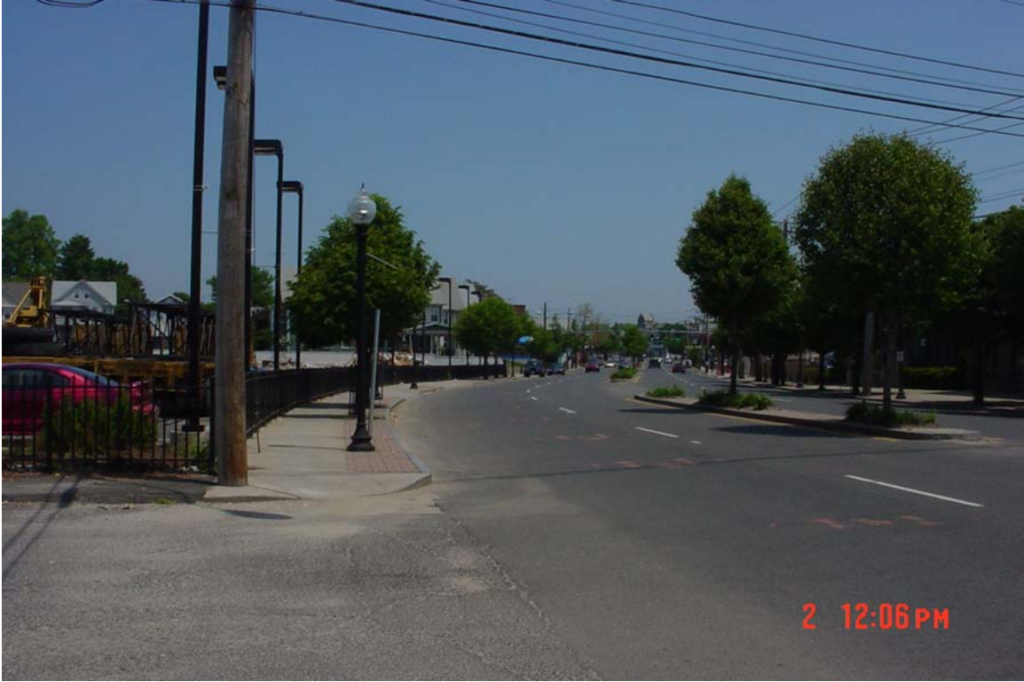
Photo 1. Route 130 (Fairfield Avenue) looking northeast at Poland Street.
