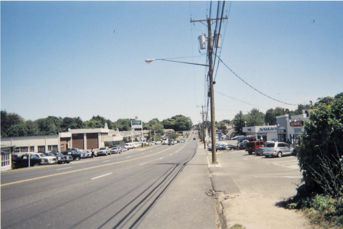
Photo 13. Route 1 (Post Road East) looking eastbound east of Crescent Street.
