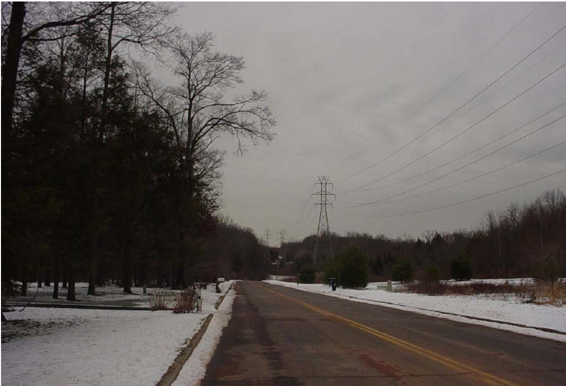
Photo 5: Old Farms Road (Cheshire) at approx. Sta. 46+00, looking southeast.
