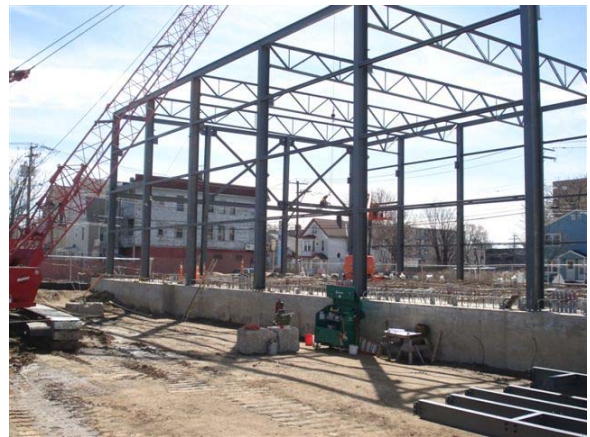
Erection of structural steel for GIS building
