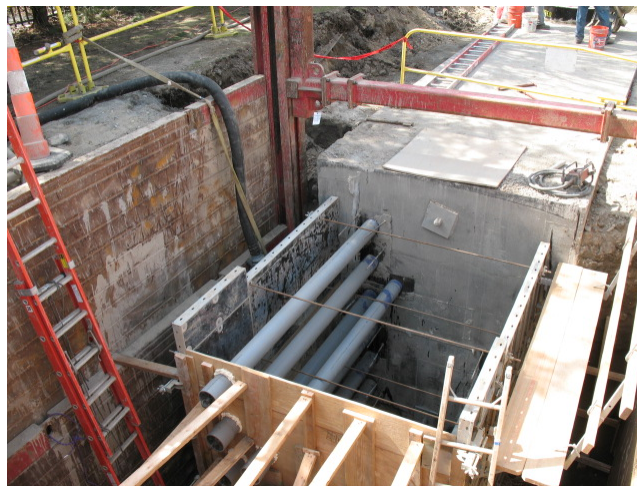
115kV Duct Bank Installation to Pequonnock Substation
