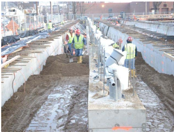
GIS building foundation in fill
