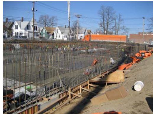
Rebar installation and concrete pouring of GIS building bottom slab.
