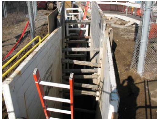
115kV Duct Bank Installation to LS Power
