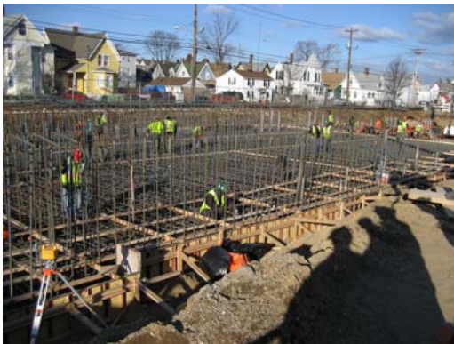
Rebar installation and concrete pouring of GIS building bottom slab.
