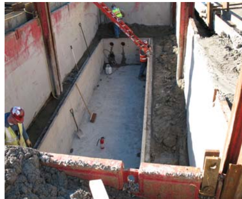
Splice Chamber 7 (Bottom half installed)
