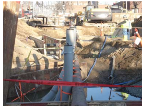
Installation of 345kV underground duct on Singer Substation site.
