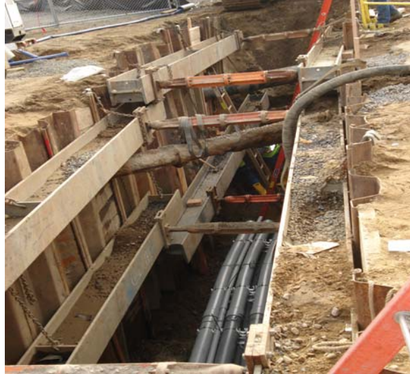
115kV Duct Bank Installation to LS Power
