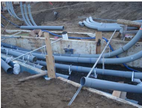
Installation of 345kV underground duct on Singer Substation site.
