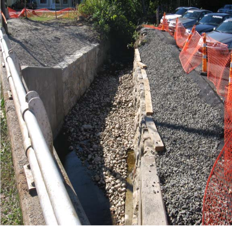
Both photographs were taken near sta. #217 at the Stony Brook crossing. Left: Hard pack on south side of stream remains moderately stable. Signs of minor migration were noted on top of the retaining wall. Right: Tree removed for construction activities remains within the parking area to the north of Stony Brook. Remove and properly dispose of if property owner has not requested for it to remain.
