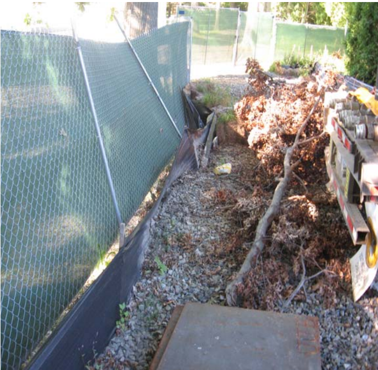
Both photographs were taken within the Sherwood Island lay-down yard. Left: Down limb located near the rear of the yard was removed from the erosion controls. Erosion controls continue to function properly. Right: Fluid filled equipment was being stored on exposed soil in an uncontained/unprotected location.
