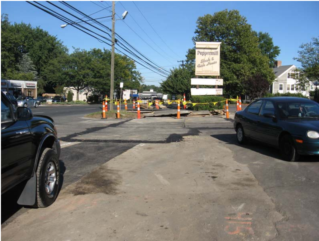
Photograph of trenching activities at and adjacent to vault #25.
