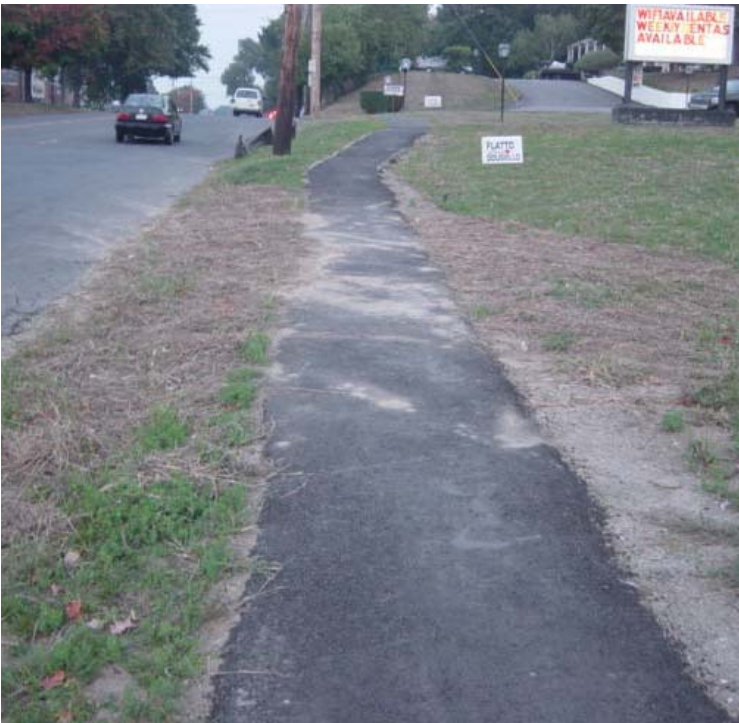
Ruts along the roadway in front of the Fairfield Inn have been stabilized with hay mulch.
