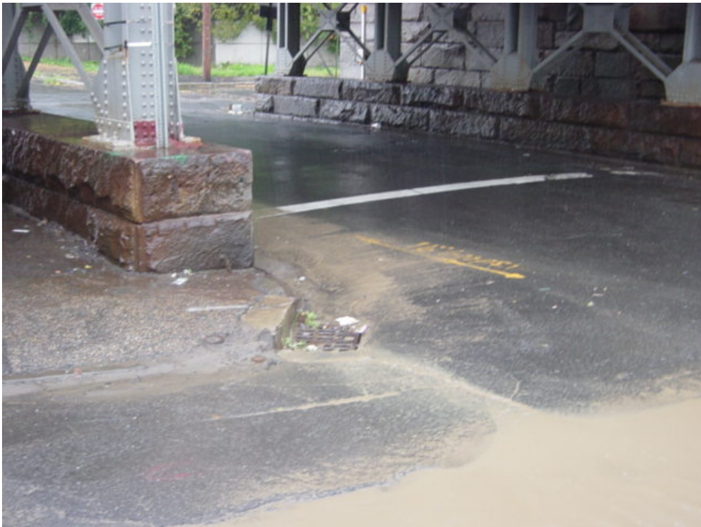
Both photographs show stormwater leaving the lay-down yard at the intersection of Railroad and Myrtle Ave. The yard is not related to this portion of the project, it appears to be part of the Glenbrook Cable portion of the project. Above: Sediment laden stormwater travels from the yard down the edge of the roadway. Below: Sediment laden stormwater (shown above) is entering an unprotected catch basin on Railroad Ave (far left of above photograph).
