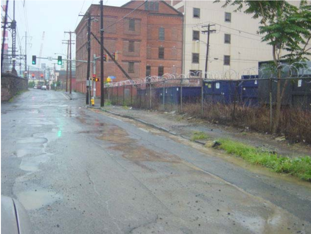
Both photographs show stormwater leaving the lay-down yard at the intersection of Railroad and Myrtle Ave. The yard is not related to this portion of the project, it appears to be part of the Glenbrook Cable portion of the project. Above: Sediment laden stormwater travels from the yard down the edge of the roadway. Below: Sediment laden stormwater (shown above) is entering an unprotected catch basin on Railroad Ave (far left of above photograph).
