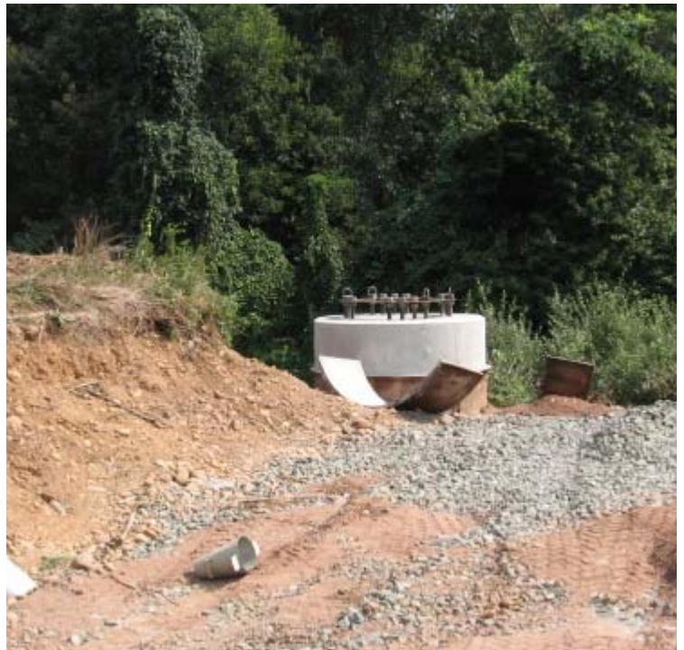
Willow St. (Hamden): Structure #4011 has been installed.
