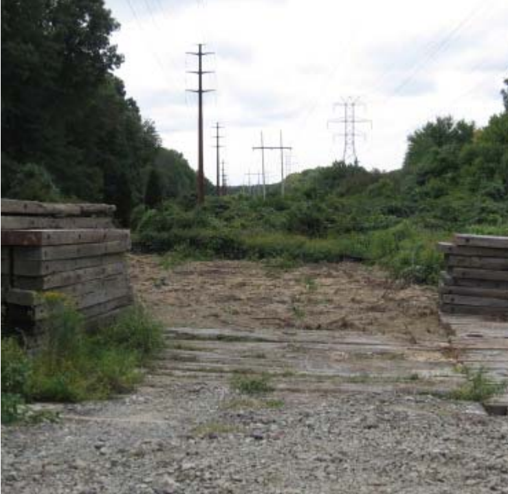
Racebrook Rd (Orange): Exposed soils from pad reclamation activities have been temporarily stabilized with mulch.
