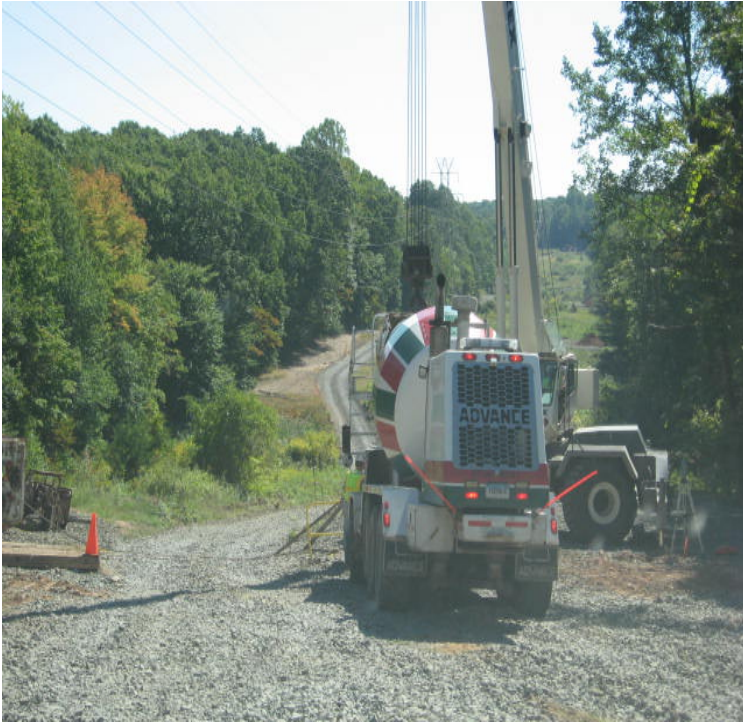
Tuttle Ave: Concrete was being poured here this week.
