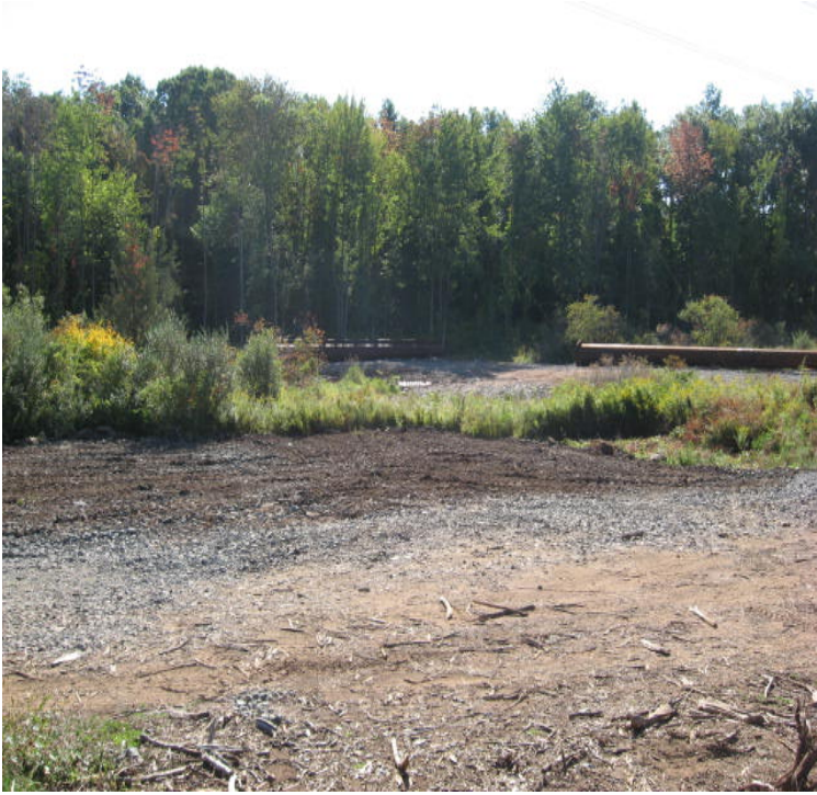
Carpenter Ln: View of the new staging area within the wetlands.
