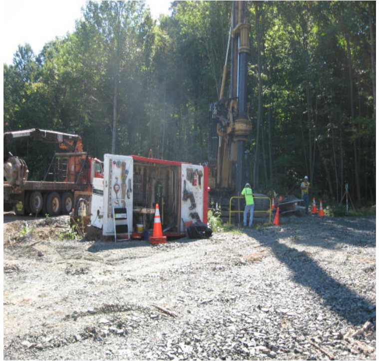
Tuttle Ave: Foundation drilling continues.
