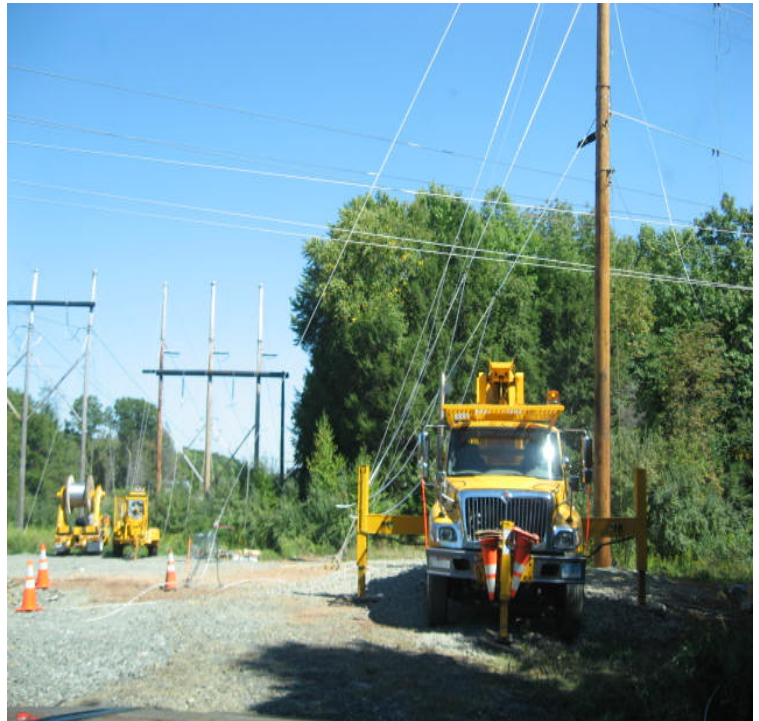
Old Farms Rd: Line pulling equipment is onsite.
