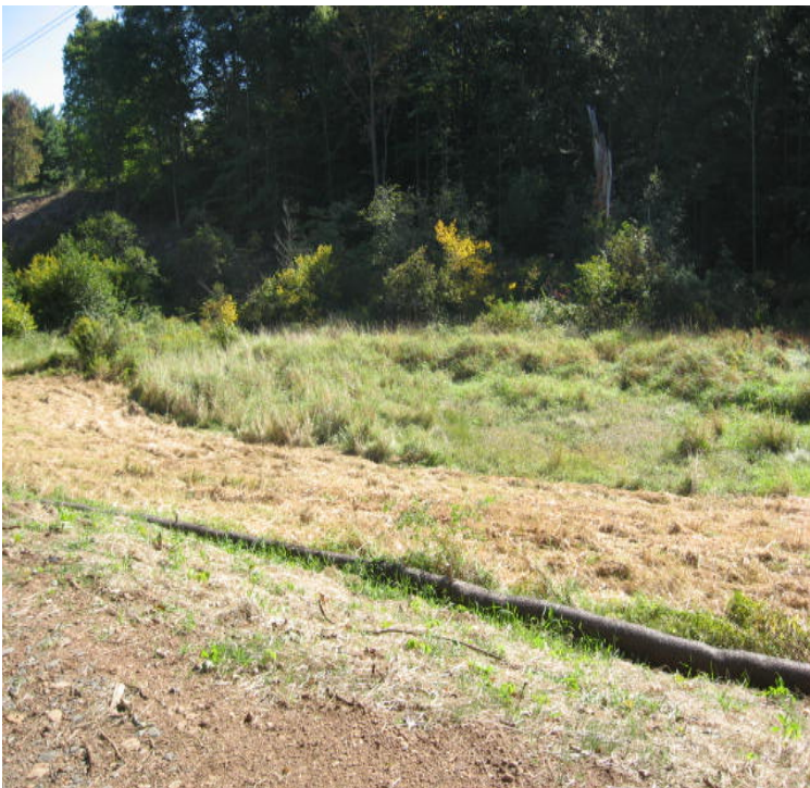
Liney Hall Ln: Fiber rolls remain in place here. Area around pool (amphibian breeding habitat) has been mowed
