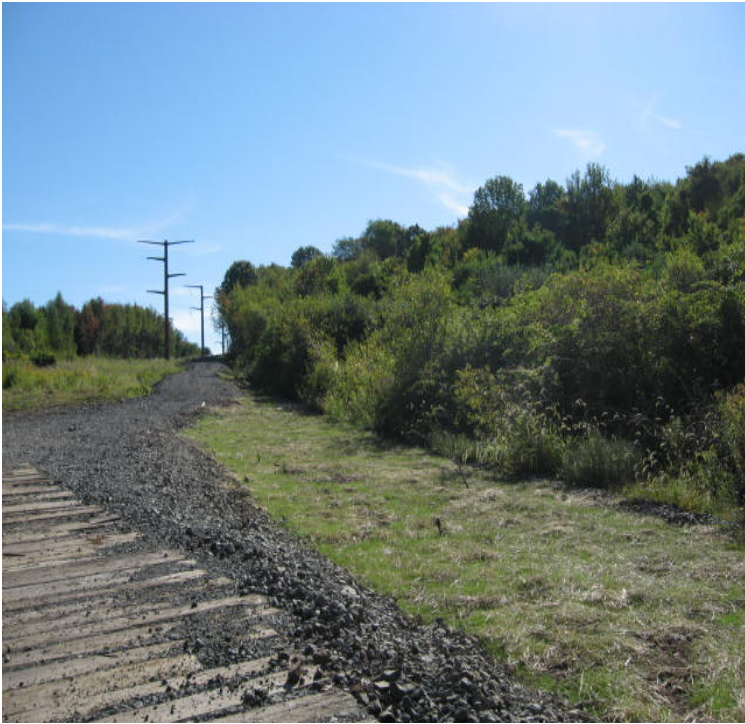
A section of the access road has been removed at Route 17 east. The disturbed area along the road was regraded, mulched, and seeded.
