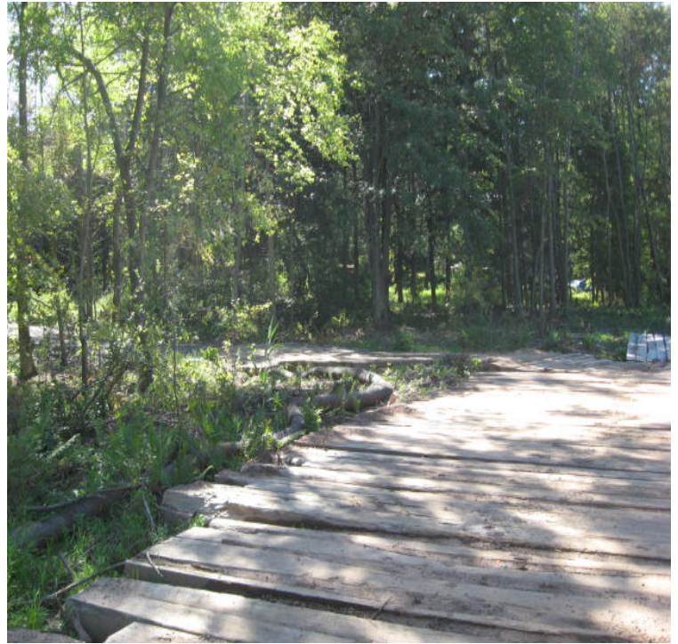
Timber mats were cleaned near structure #24580, but some sediment was swept over the controls and into the wetland in this section.
