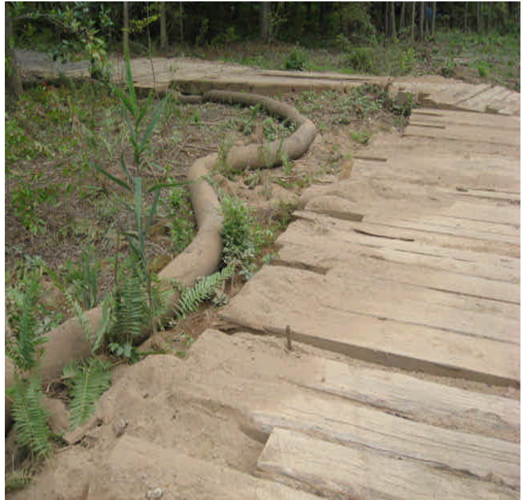
Timber mats were cleaned. However, some of the sediment has migrated to the controls and edge of the mat within the wetland.
