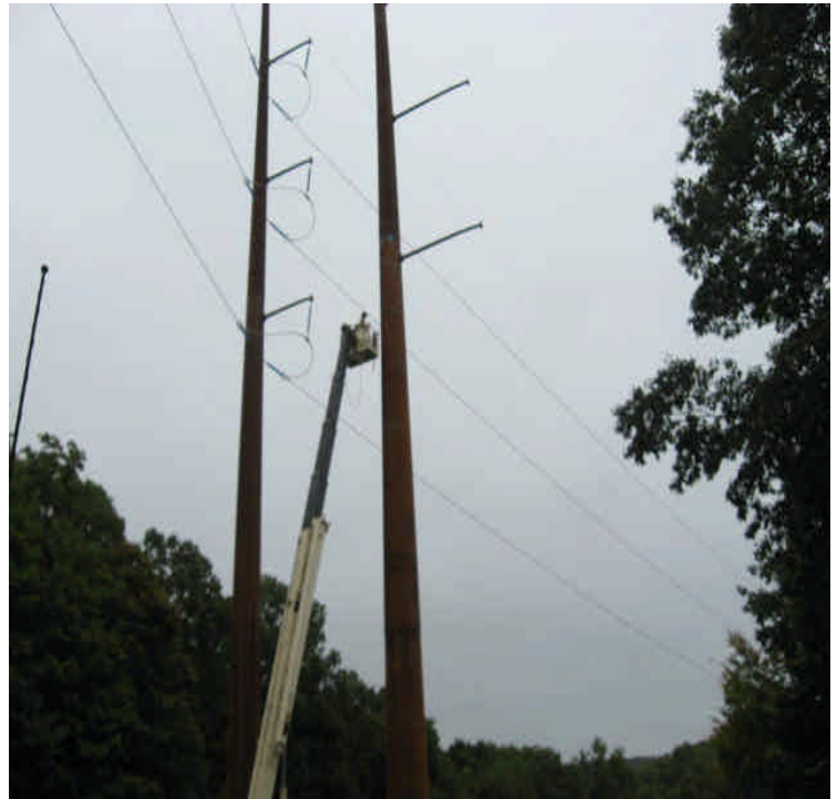
Black Walnut Dr: Crews were performing wire work; Installing pull boxes.
