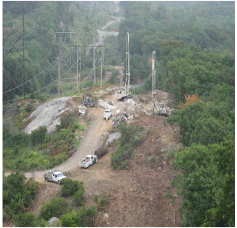
Shunpike Rd: View of drilling and foundation installation.
