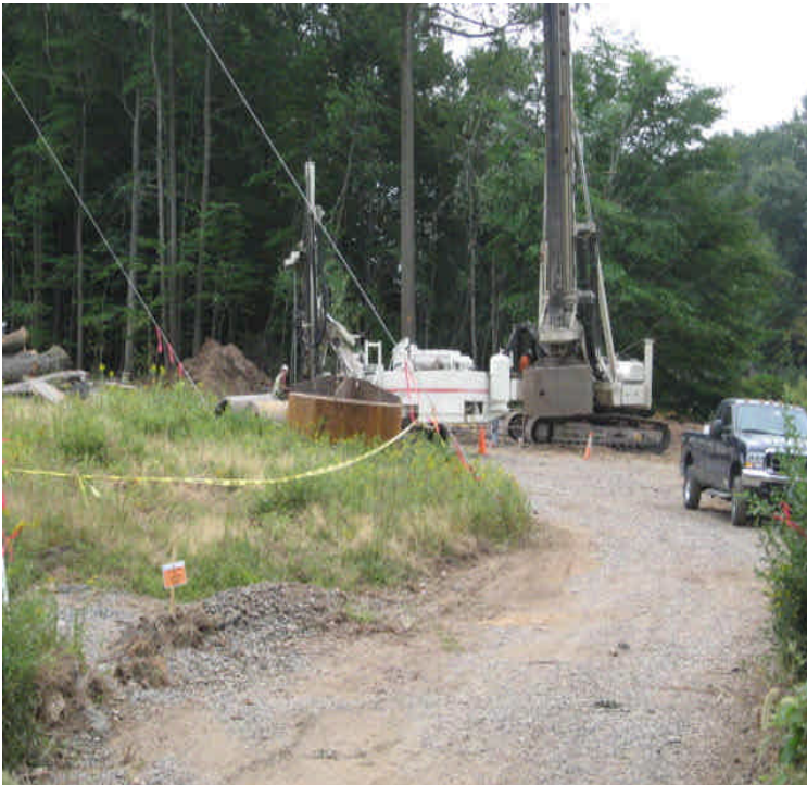
Bartholomew Rd: Crews were drilling a new foundation.
