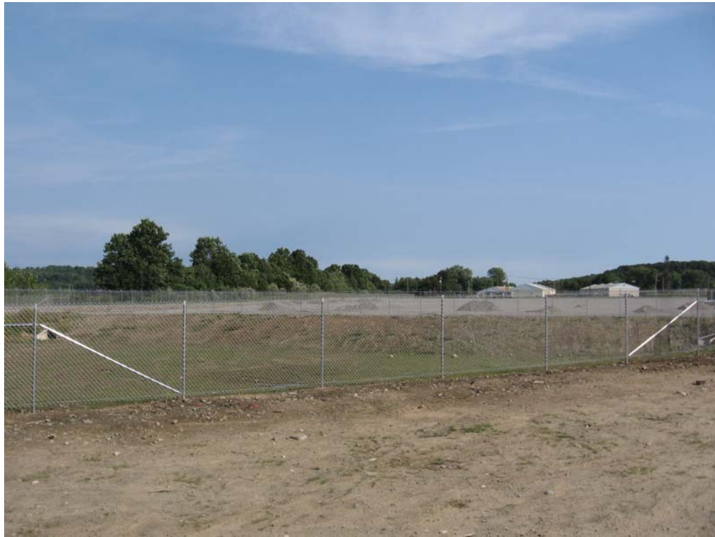
A view of the Substation site from the southern boundary.
