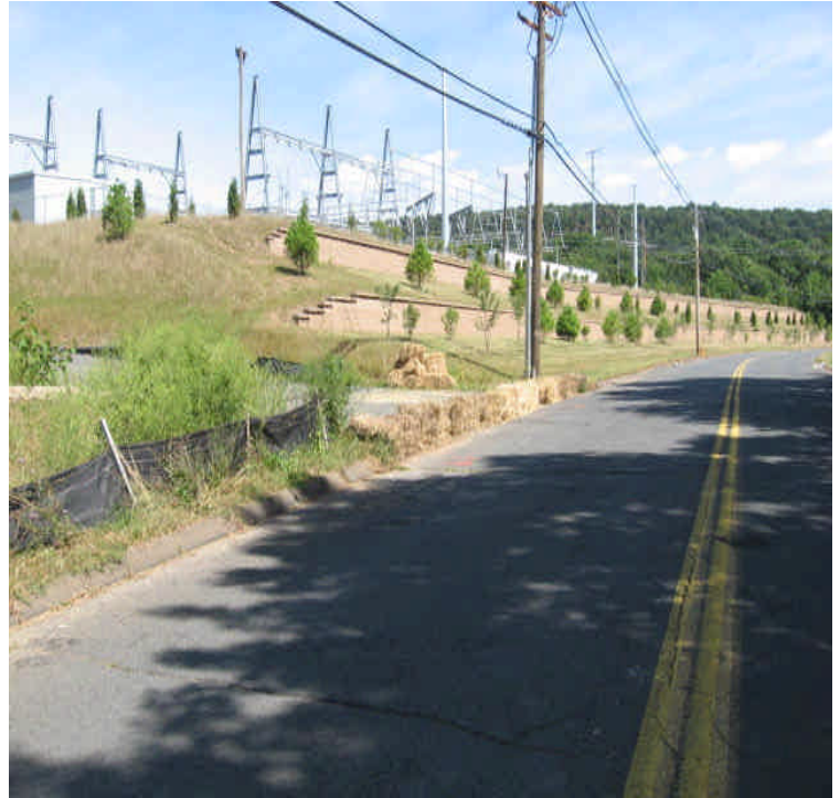
Haybales remain in place across the western site access drive.
