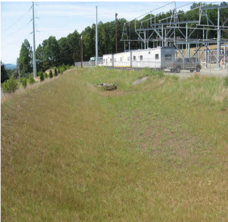
View of the detention basin and sediment trap. Vegetative cover was well established
