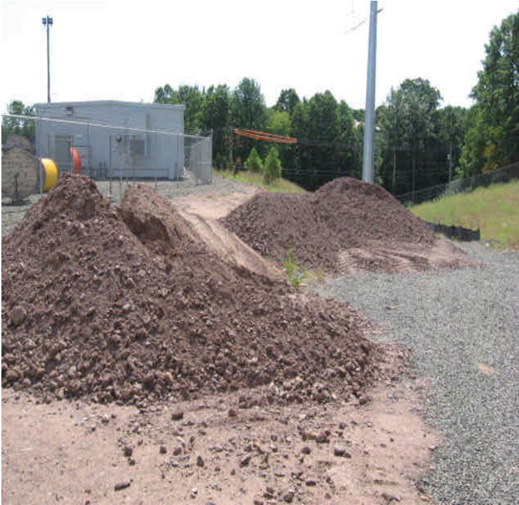
A view of stockpiles along the western access road.
