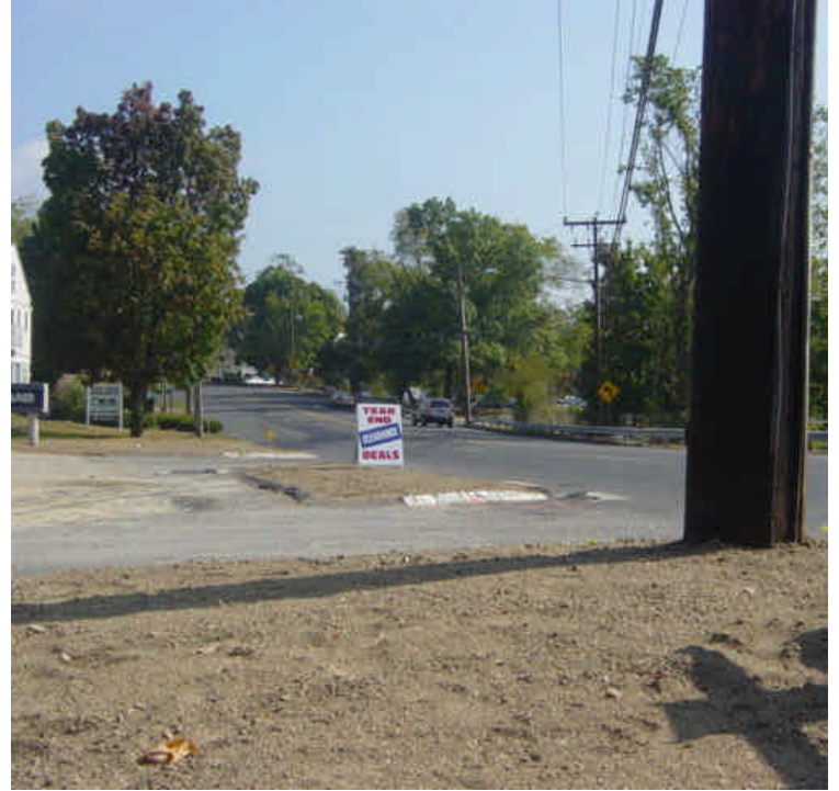
Both photos were taken at sta. #217 (Stony Brook). Left: Erosion controls remain between the hard-pack material and the brook. Right: Exposed soil has been seeded but mulch is recommended for stabilization.
