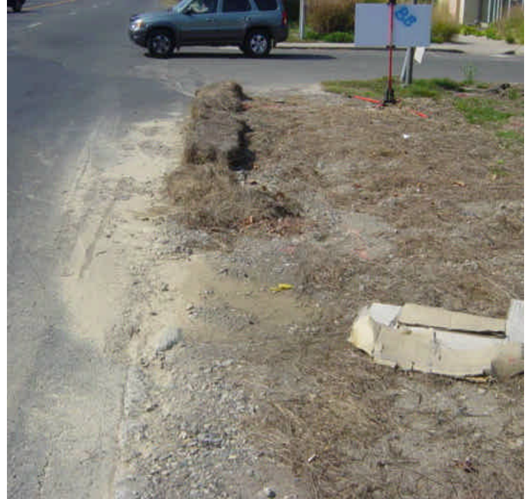
A minor amount of sediment from run-off was visible along the curb near sta. #838 (vault #23), which was previously covered with hard-pack and stabilized with hay mulch. Sweep roadway as necessary. Continue restoration/stabilization efforts and monitor until area is permanently stabilized.
