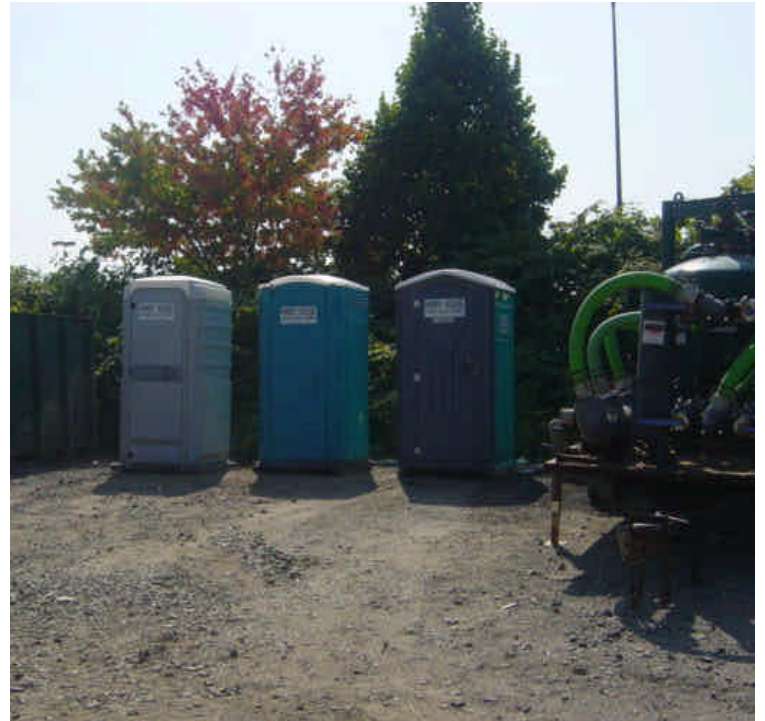
Portable sanitary facilities at the King's Highway lay-down yard were relocated away from the nearby watercourse.
