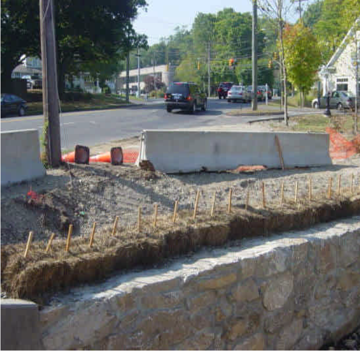
Both photos were taken at sta. #217 (Stony Brook). Left: Erosion controls remain between the hard-pack material and the brook. Right: Exposed soil has been seeded but mulch is recommended for stabilization.
