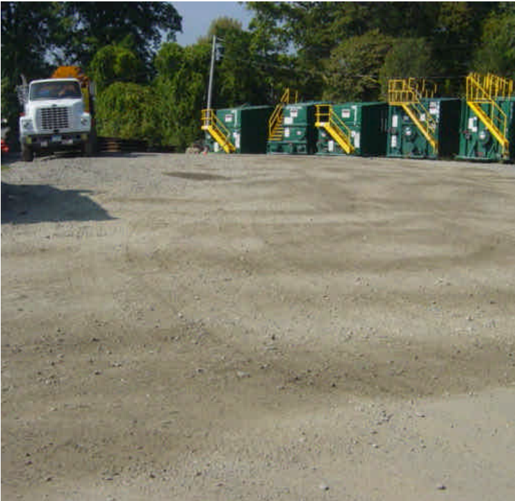
The Sherwood Island lay-down yard was recently watered down in an effort to control airborne dust migration.
