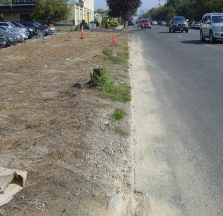
A minor amount of sediment from run-off was visible along the curb near sta. #838 (vault #23), which was previously covered with hard-pack and stabilized with hay mulch. Sweep roadway as necessary. Continue restoration/stabilization efforts and monitor until area is permanently stabilized.
