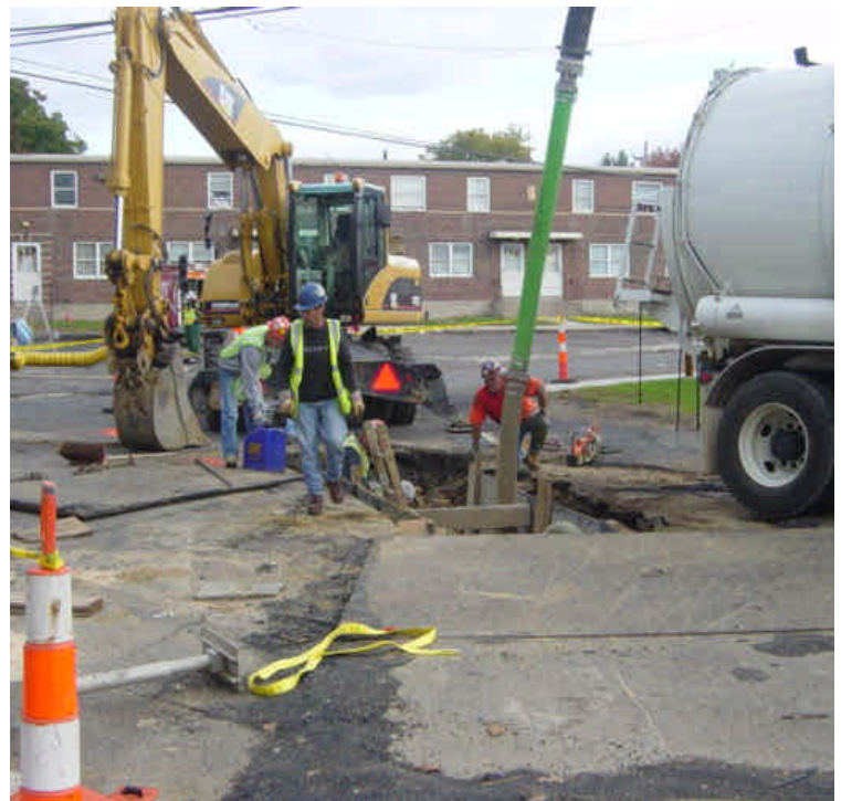
Trenching and backfill work continues near sta. #771-#772.
