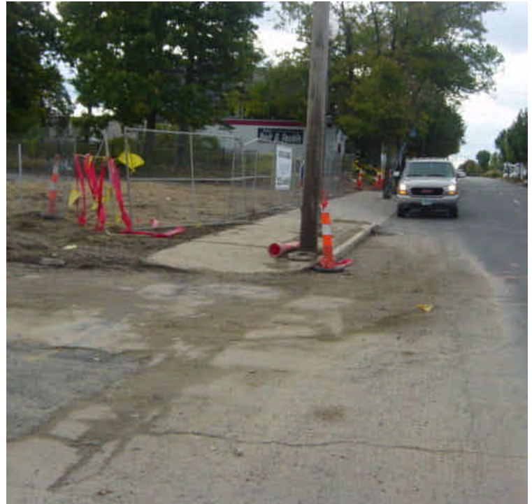
Heavy sediment accumulation near sta. #695 (vault #42) was observed along the shoulder and sidewalk areas. The source of the accumulation was unclear but may have been generated by the placement of a temporary stockpile in this area during a previous workday. Sweep roadway and provide permanent restoration efforts in this area.
