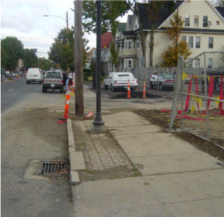
Heavy sediment accumulation near sta. #695 (vault #42) was observed along the shoulder and sidewalk areas. The source of the accumulation was unclear but may have been generated by the placement of a temporary stockpile in this area during a previous workday. Sweep roadway and provide permanent restoration efforts in this area.
