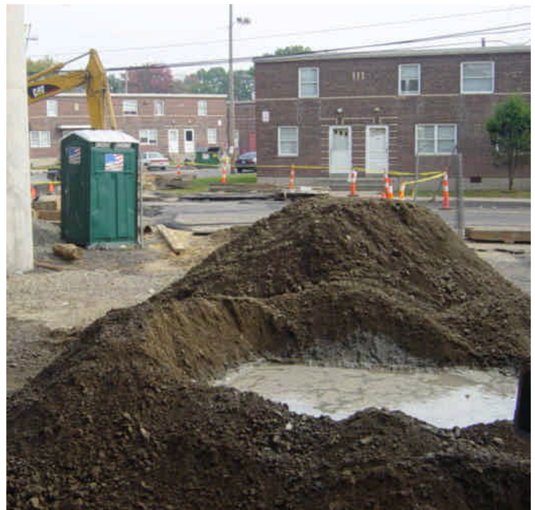
Trenching and backfill work continues near sta. #771-#772 (left). A small, designated concrete washout area was observed near sta. #771-#772 (right). The area was contained, but the slurry eventually needs be removed and properly disposed of.
