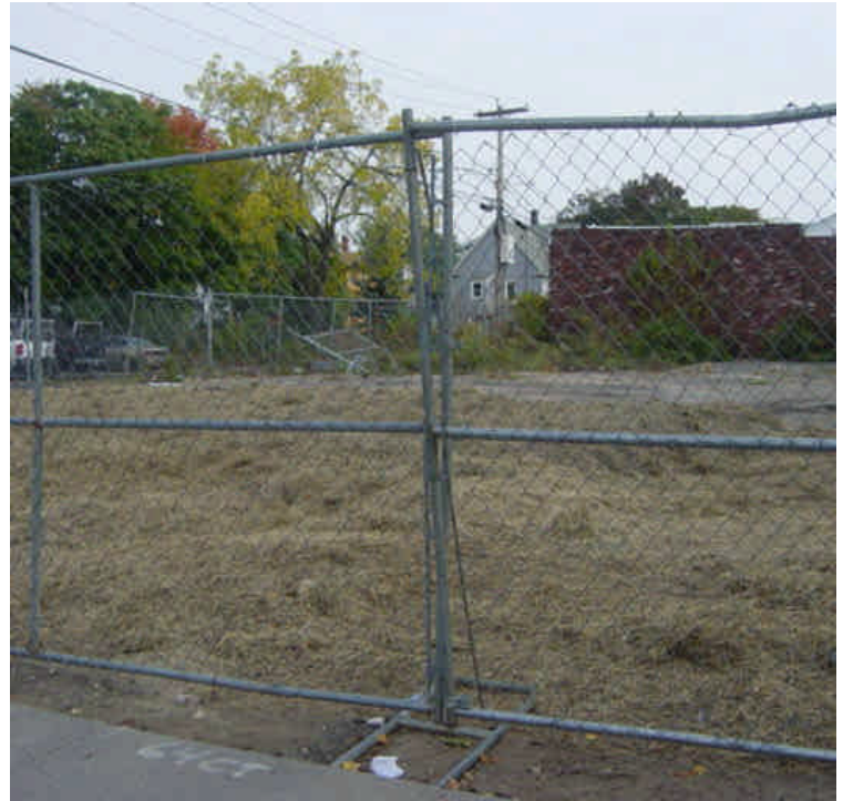
Hay mulch has been applied over the exposed soils near sta. #695. Permanent restoration efforts will be necessary in this area.
